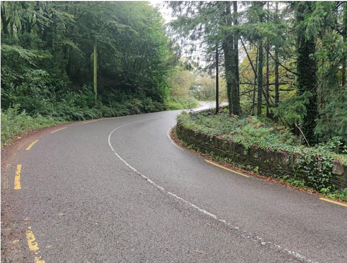
Photo 4.1: Existing R605 Road Layout
