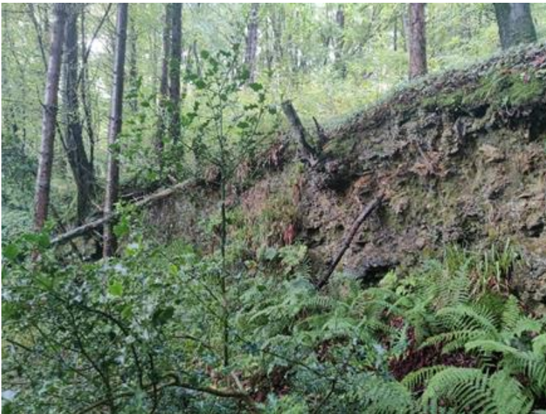
Photo 4.3: Exposed Earth Banks Within Woodland
