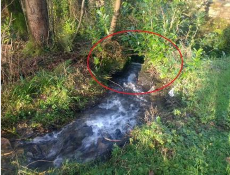
Photo 4.8: Stream and Top of Weir (Circled)
