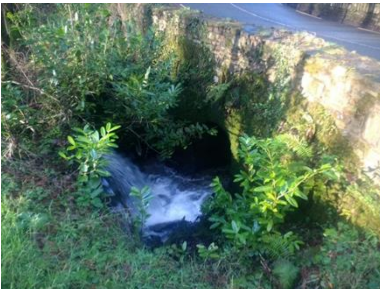
Photo 4.9: Culvert face and Stream Immediately Downstream of Weir
