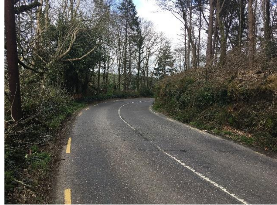
Figure 9 View looking North along R605 with outcrop on the right and tight bend
