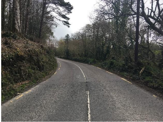
Figure 8 View looking South along R605 with rock outcrop on the left
