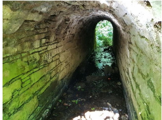
Figure 5 View looking towards River Bandon (West) from the inside of the existing culvert
