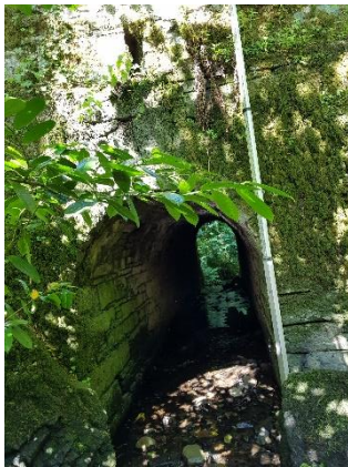
Figure 10 View of the existing culvert
