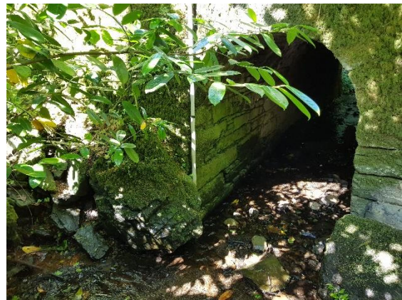
Figure 11 View of the existing culvert
