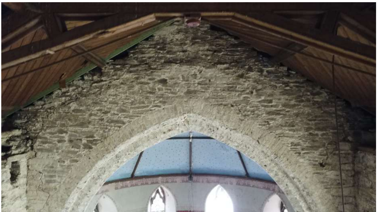
• Fig 60. Roof underside and arch over altar, with signs of movement to left and mid span.
