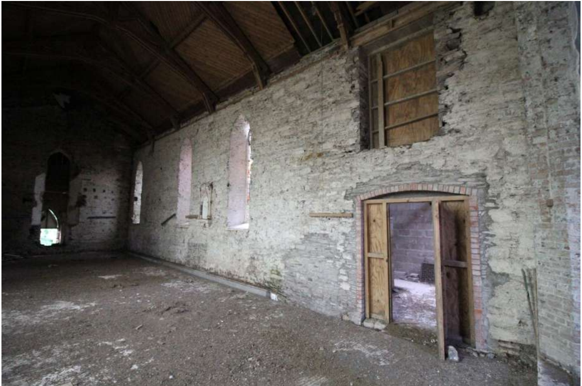
• Fig 50. Inner North wall with stripped plaster and new opes.
