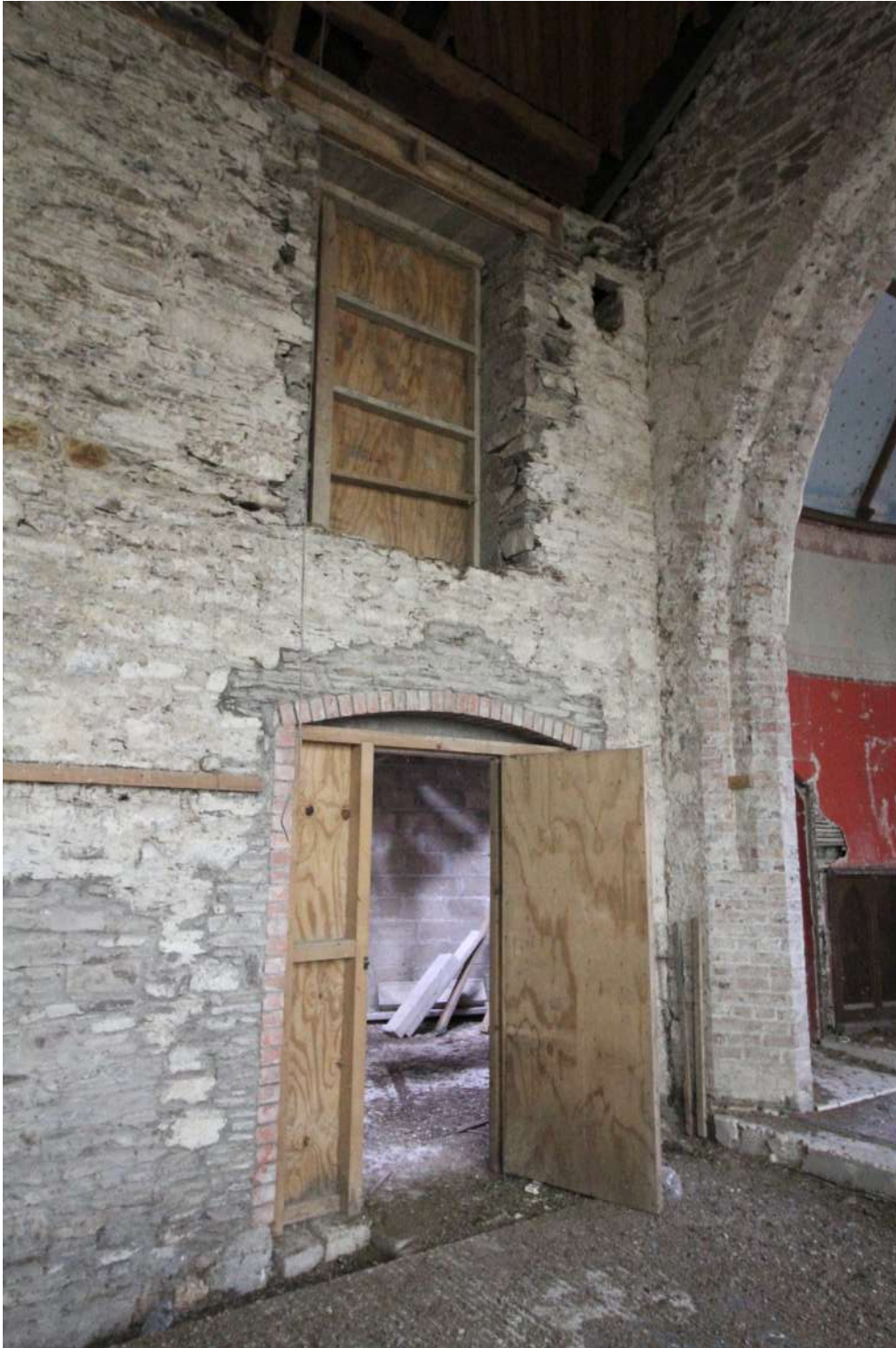
• Fig 49. New opes formed in North wall forming access to Annex.
