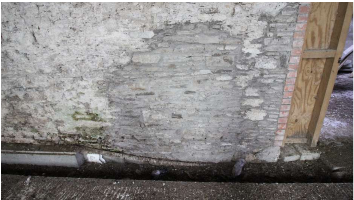
• Fig 62. Perimeter 'duct' left around new RC floor around church. Indication of some minimal insulation.
