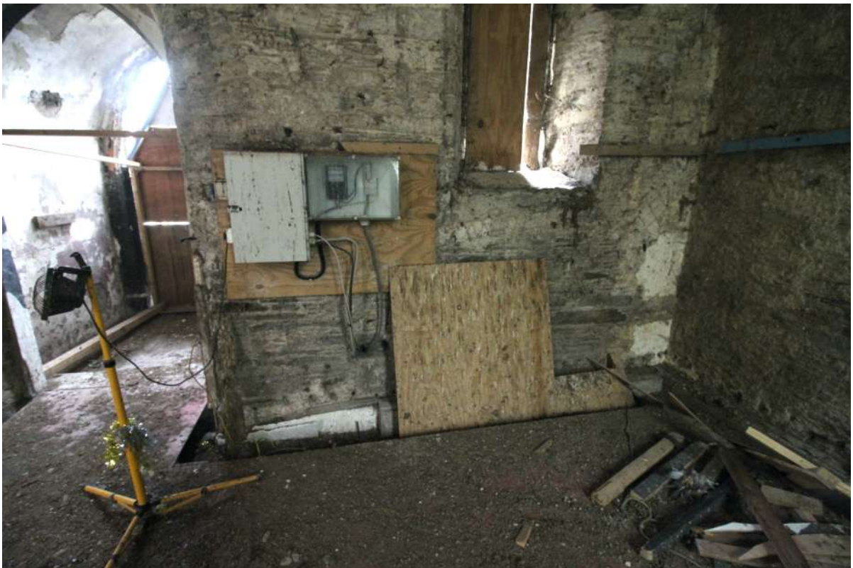
• Fig 58. Looking South alongside entrance lobby, with temporary ESB supply panel.
