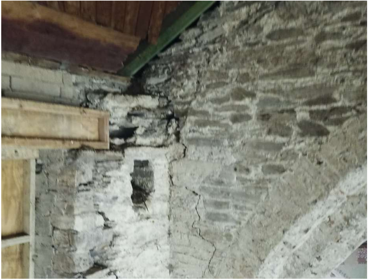
• Fig 61. Signs of movement to left of arch span.
