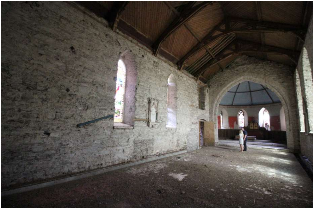
• Fig 51. Inner North wall with stripped plaster and new opes.
