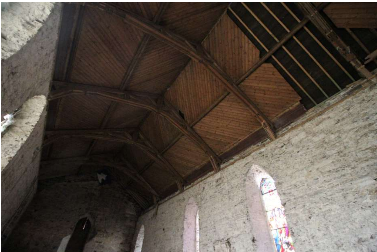
• Fig 56. Panelled ceiling and exposed roof trusses.
