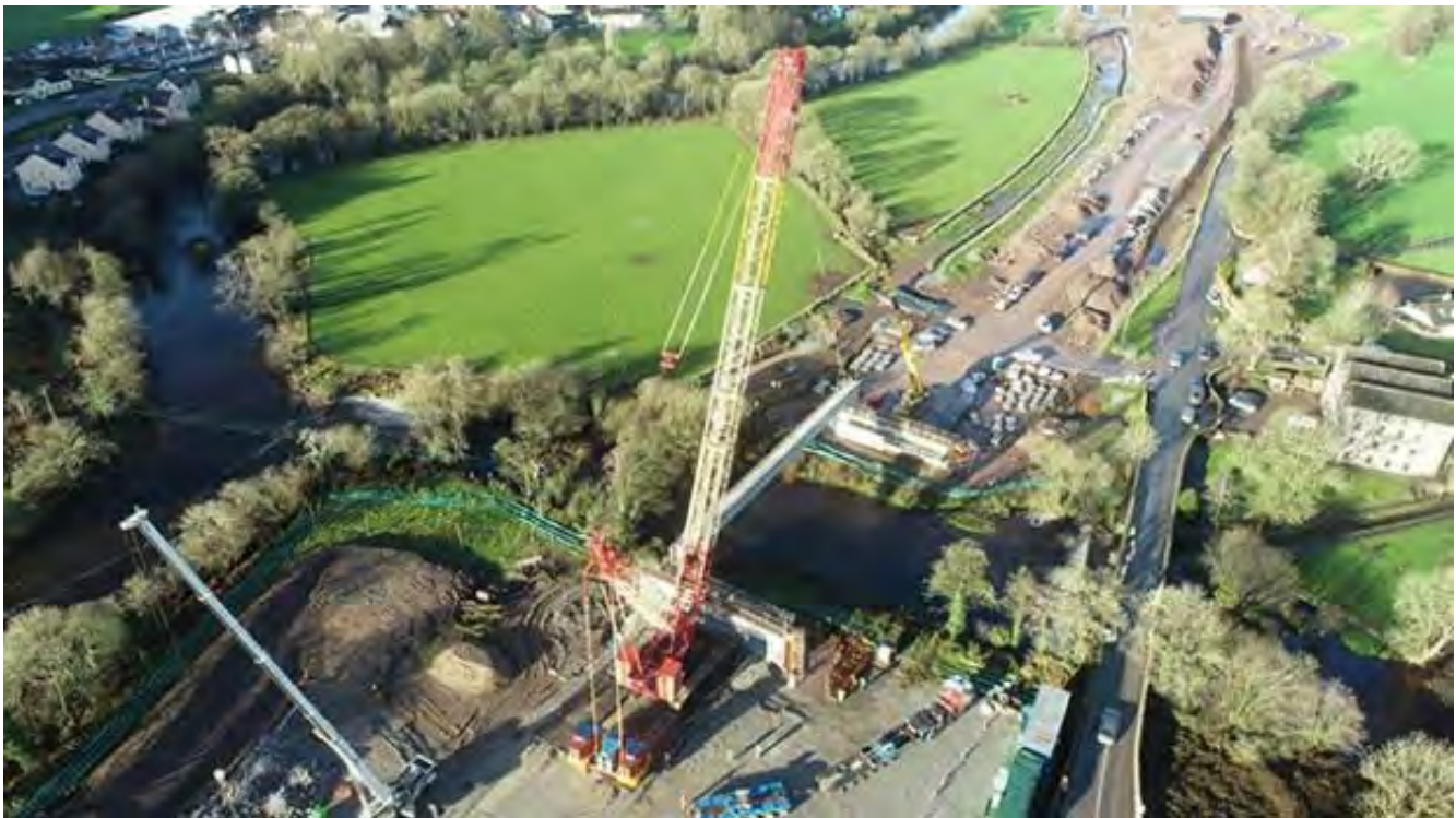
Figure 4.3: Contractors working on the N22 Baile Bhuirne Macroom by-pass
