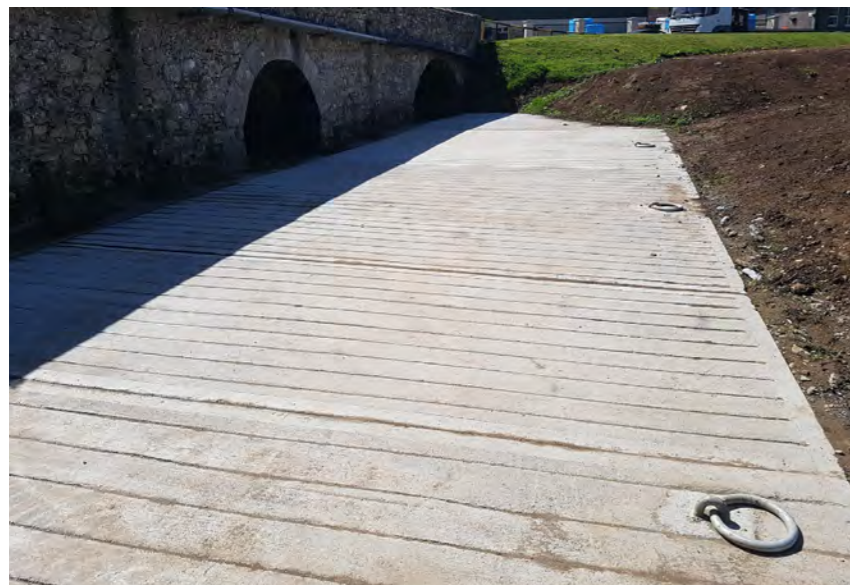
Blueway Access Concrete Plinth
