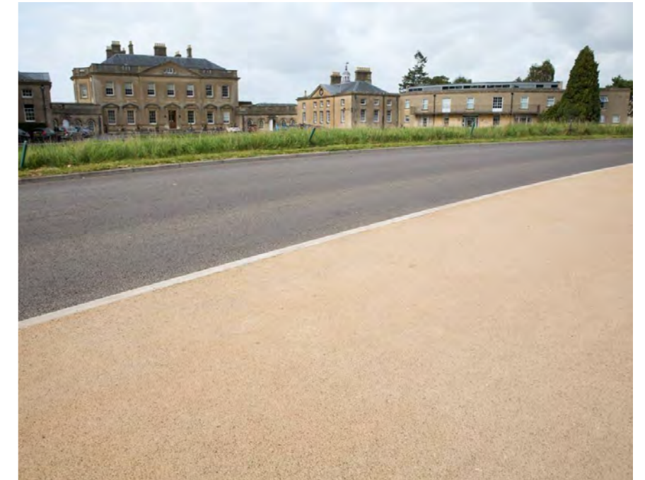
Buff Tarmacadam Road in Heritage Landscape
