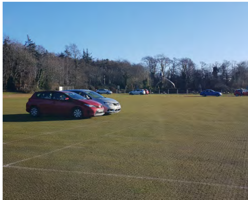
Reinforced Grass Overflow Parking & Pathways in Town Park
