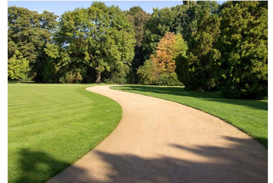
Breedon Gravel Pathway with Steel Edging
