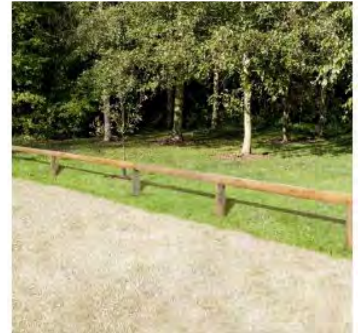
Timber Knee Railing in Demesne Landscape
