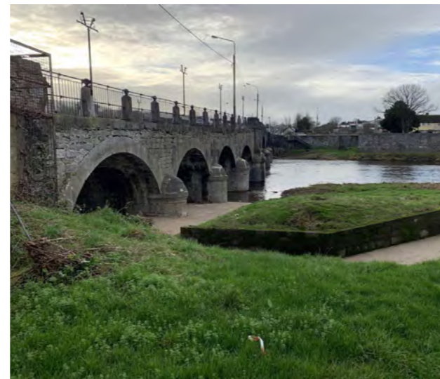
River Arch Bridge
