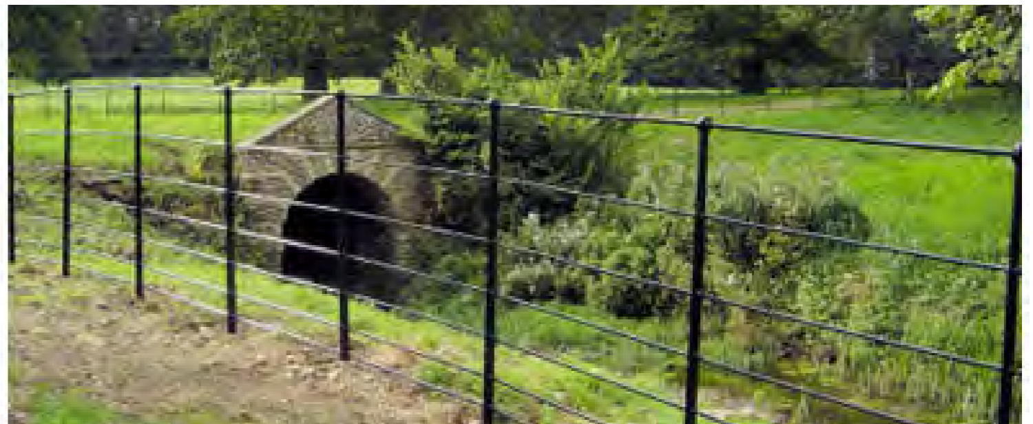
Estate Railing in Castle Grounds
