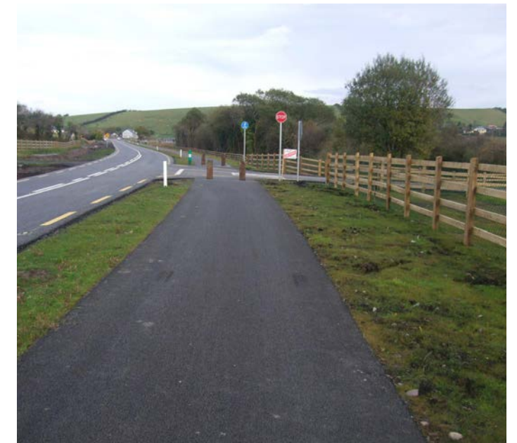
Figure 18.1 Cycle Track alongside the N59 at Newport, County Mayo
