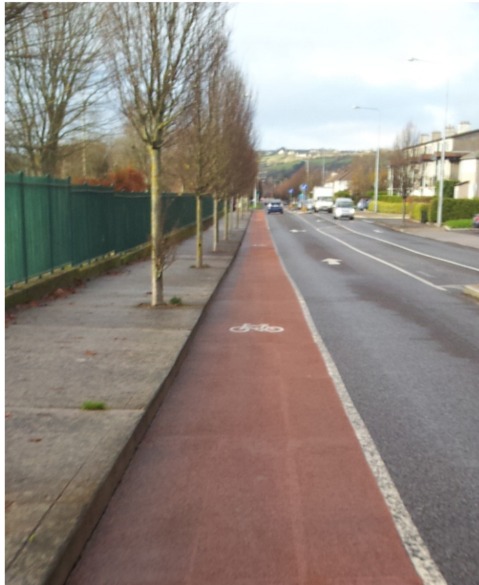
Figure 8.1 Existing cycle lane at Clashduv Road
