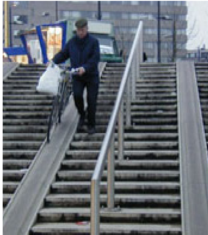
Figure 7.6' Example of wheel ramp for cyclists to push bike up or down steps
