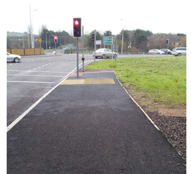
Figure 3.14 New at grade crossing at Sarsfield Roundabout
