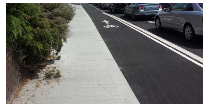
Figure 7.4 Segregated Cycle Track Retrofitted to Urban Dual Carriageway
