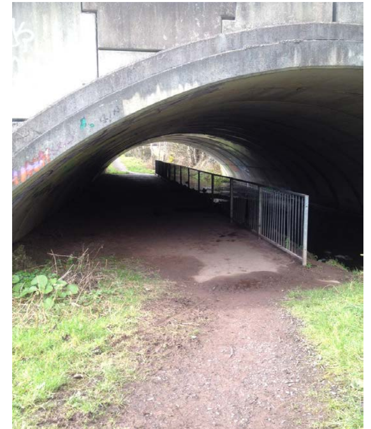
Figure 8.3 Example of underpass along existing route south of N40.
