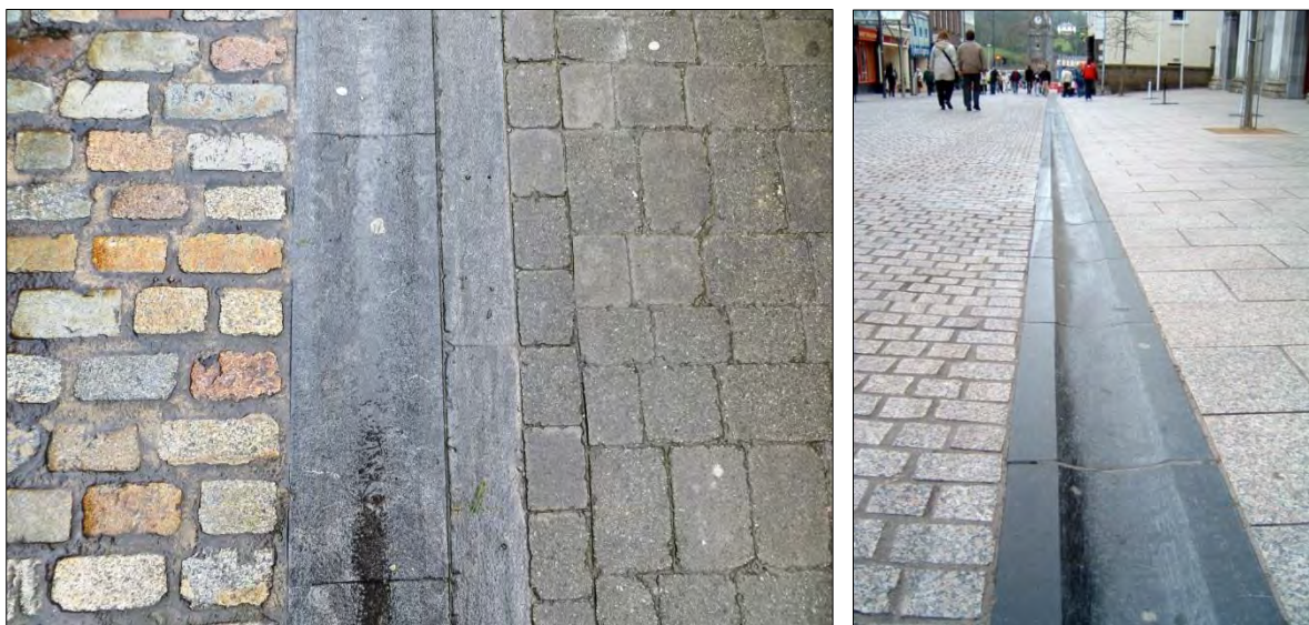
Figure 6.16 Detail of Cobble Stone Roadway, Concrete Paviors and Limestone gutter
