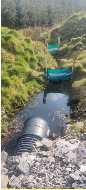
Photograph 3: Drainage ditch which is piped under hardcore and existing road.
