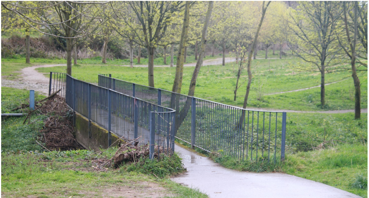
Figure 23 Mallow Town Park (Castlepark) Existing bridge crossing of Caherduggan Stream
