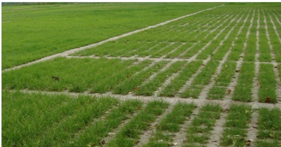
Figure 45 Reinforced grass/grasscrete surface for event parking area(reference image from Farmleigh House, Dublin).
