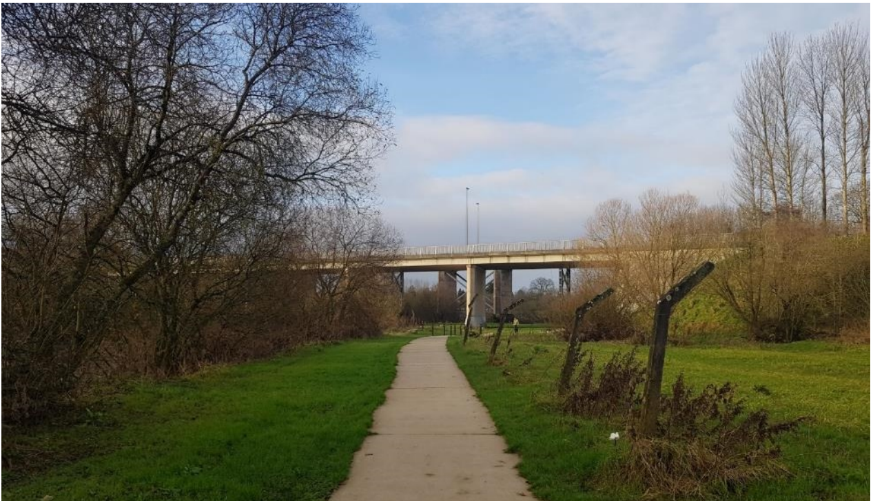
Figure 21 Mallow Town Park looking west to N20 and Railway Viaduct
