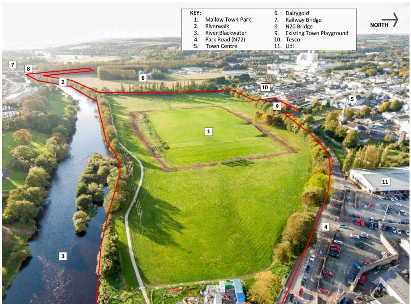
Figure 12 Site context - Mallow Town Park and Riverwalk west towards Railway Bridge
