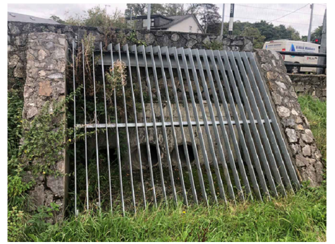
PHOTO '1' EXISTING HEADWALL AND SCREEN DETAIL AT ROADSIDE
