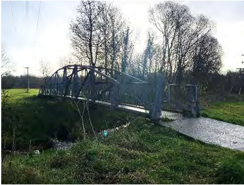
Fig. 13: Grounds south of Mallow Castle, pedestrian bridge.
