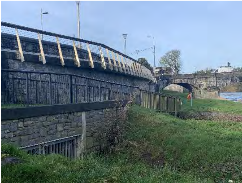
Fig. 22: Quay walls, south east of Mallow Bridge.
