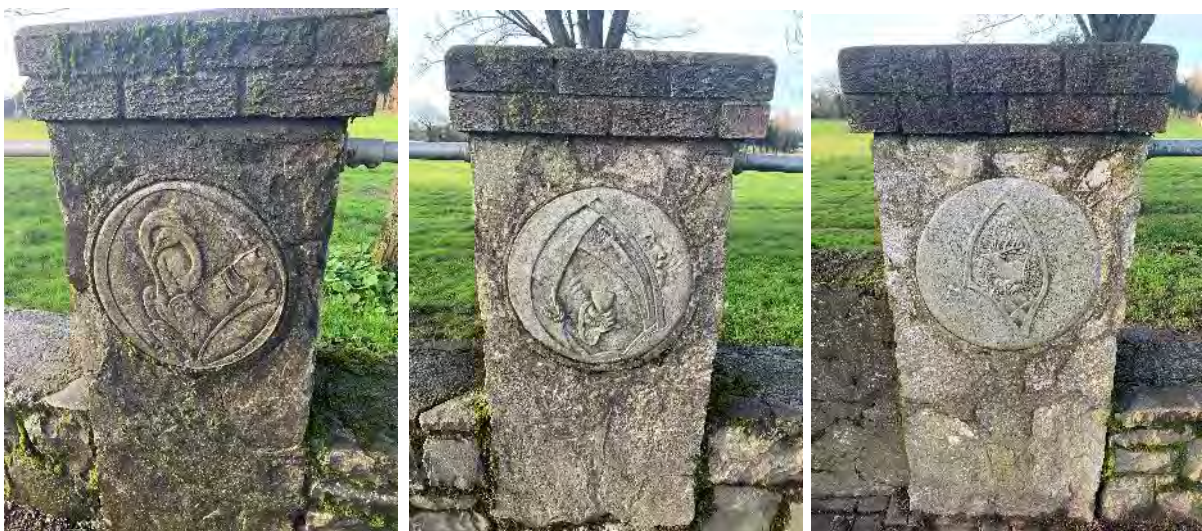
Fig. 18: Cast decorative panels to piers on the north side of the Town Park.
