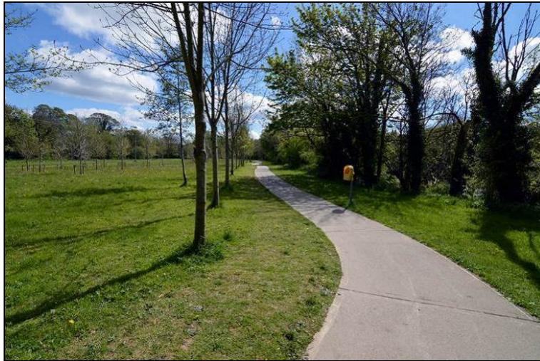
Photograph 12: Existing 2m wide concrete path on the River Walkway, looking east.
