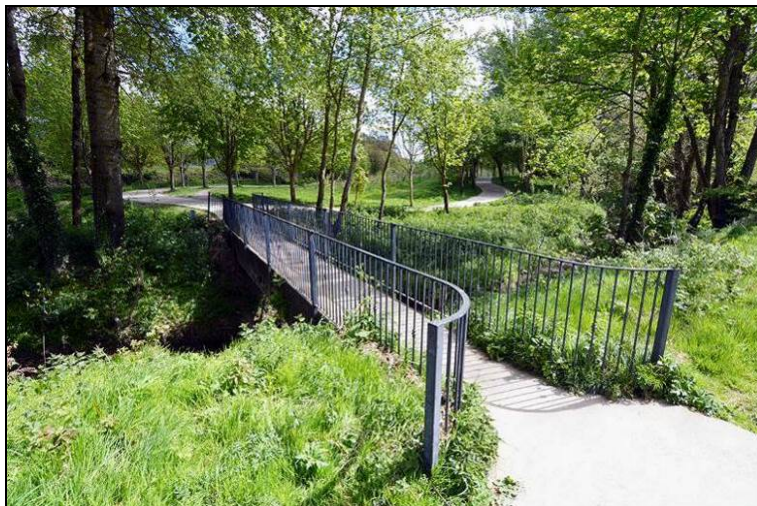
Photograph 13: Pedestrian bridge over the Caherduggan stream, to be upgraded with a wider deck, looking east.
