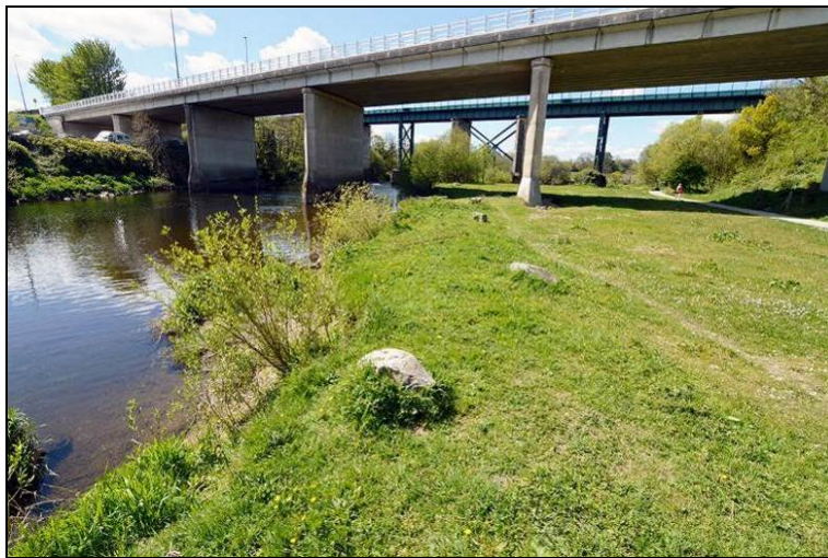
Photograph 1: Proposed grass meadow, and fishing stand location – “Ten Bridge Arch”, looking west.
