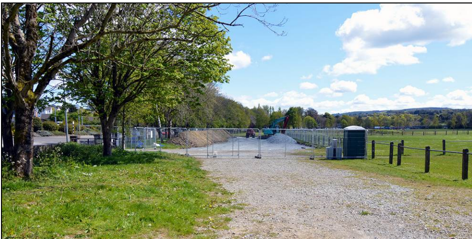
Photograph 6: View of site of the car park, now a temporary construction compound, for the upcoming Mallow Sewerage Scheme, looking east.
