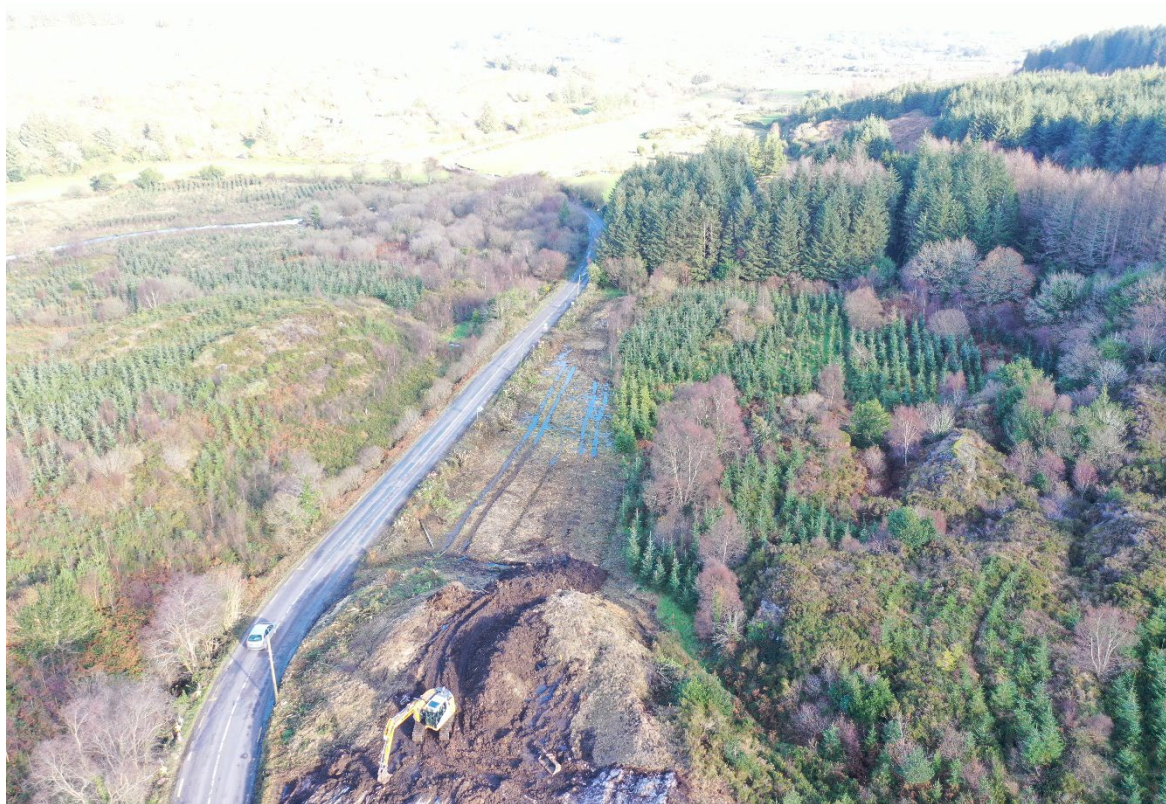
Figure 4 Aerial view looking east along the R585
