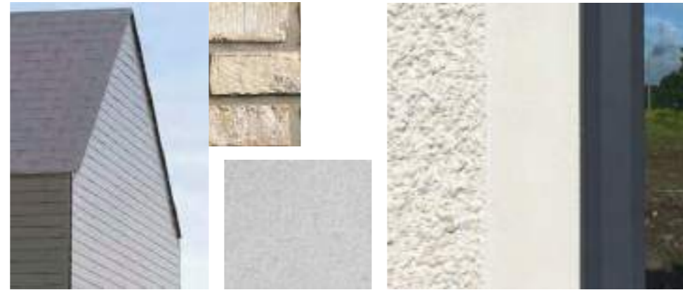
Selection of vernacular materials, including slate, brick, smooth render and textured render
