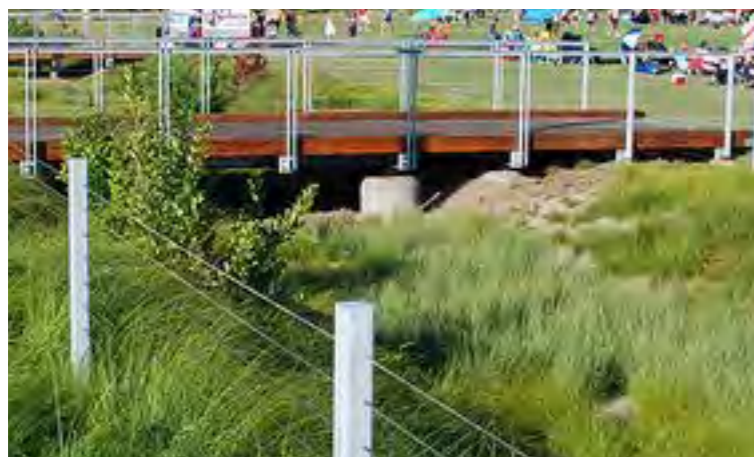
Pedestrian bridge over watercourse
