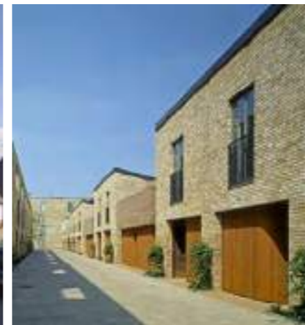
Integrated garage parking Ref: Accordia, Cambridge, FCB Studios
