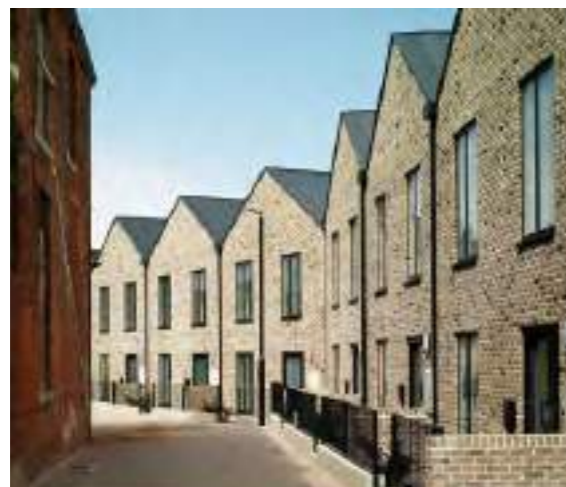
Contemporary development with high quality materials and roofscape Ref: Kelly's Avenue and Stable Lane, Dún Laoghaire-Rathdown County Council
