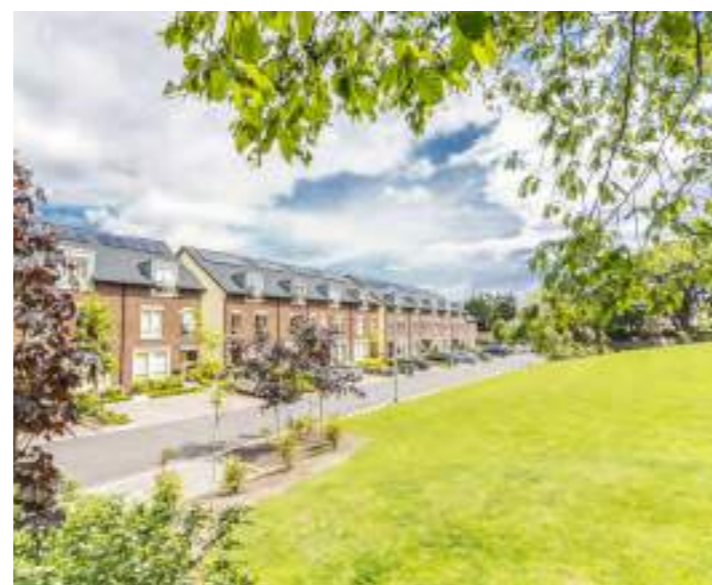
Public realm overlooked by 3 storey houses Ref: Honey Park, Dún Laoghaire, McCrossan O'Rourke Manning
