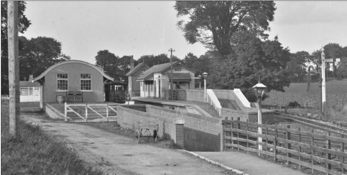
Figure 3: Historic photograph of Carrigaline railway station c. 1900 (Source: National Library of Ireland) – this former railway station is located approximately 400 metres to the south-south-west of the proposed Bridgemount Link
