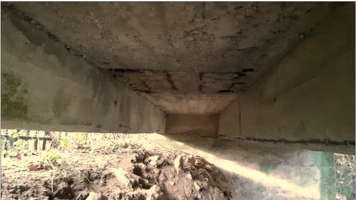
Plate 3: Underside of overpass looking west
