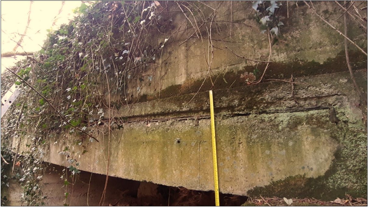
Plate 2: Northern elevation of overpass
