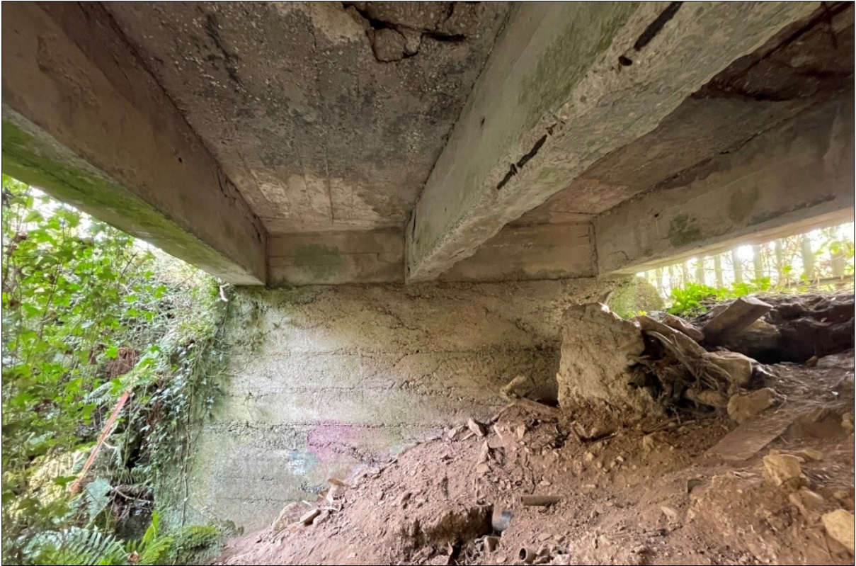
Plate 4: Underside of overpass looking east
