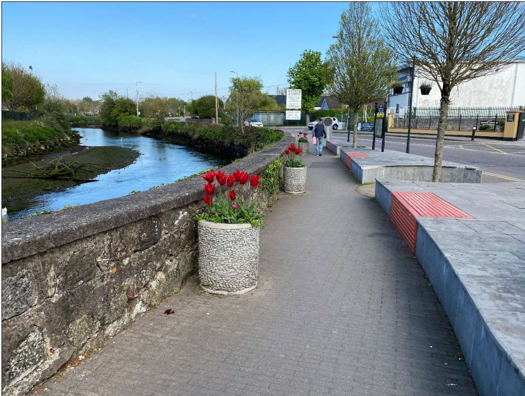
Plate 7: Random rubble wall and seating area on the northern side of R612
