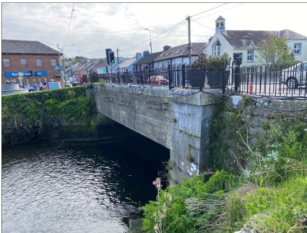
Plate 6: Carrigaline Bridge (CHS 3) over Owenboy River along Main Street
