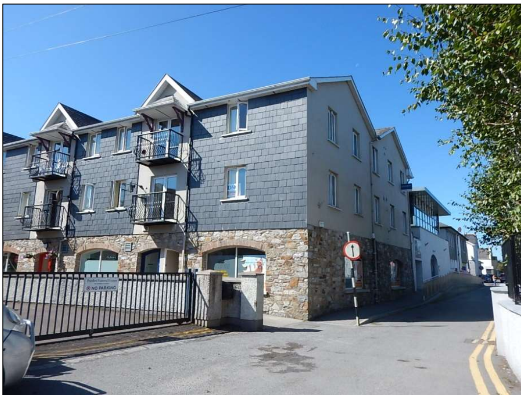
Plate 5: Former flour mill (CO087-033; PS 00579), now converted into apartments
