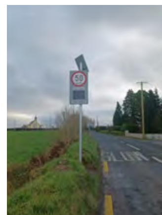
Completed speed safety signage at Ballydaly
