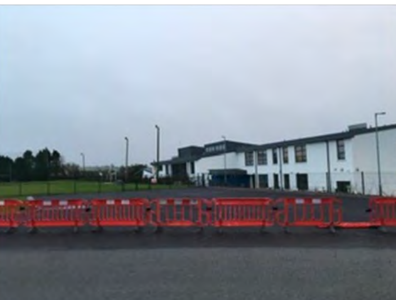
Works to set down area in Clondrohid
