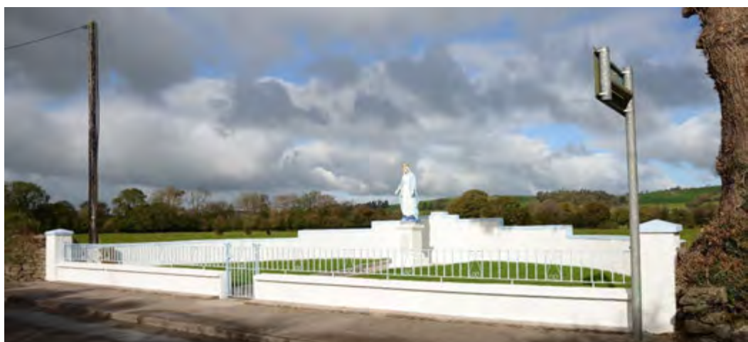
Refurishment to Crookstown Grotto
