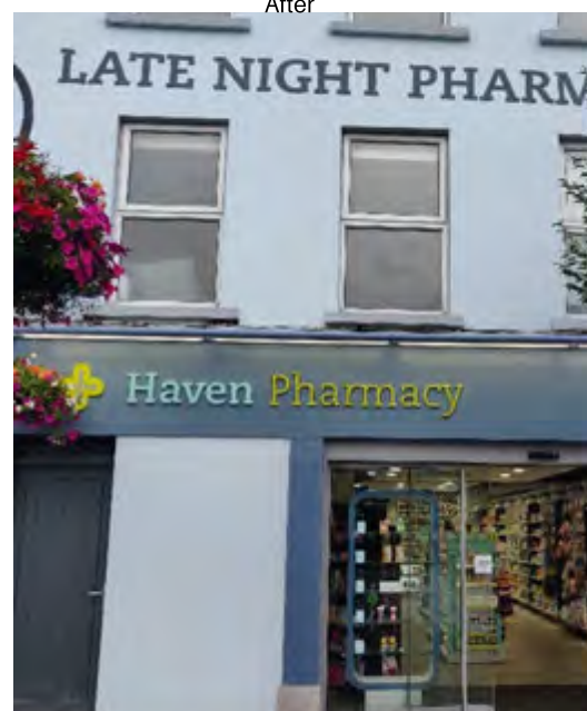
works completed at Haven Pharmacy
