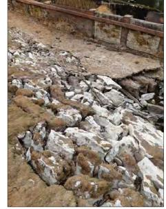
WEIR APRON DISINTEGRATED AND WASHED AWAY AT JUNCTION WITH FISH PASS
