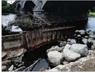
$\frac{\rm _{H}}{\rm ^{0075}} \frac{\rm VIEW~OF~TEMPORARY~REPAIRS~TO~FISH~PASS~AND}{\rm DISLODGED~MATERIAL~FROM~WEIR}$
