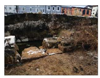
F VIEW OF DAMAGE TO FISH PASS WALL
