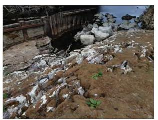
$\underbrace{ \begin{array}{c} \textbf{J} \\ \textbf{0076} \end{array} }_{\textbf{Q076}} \underbrace{ \begin{array}{c} \textbf{WEIR APRON DISINTEGRATED AND WASHED} \\ \textbf{AWAY AT JUNCTION WITH FISH PASS} \end{array} }_{\textbf{Q076}}$
