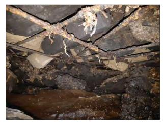
$\frac{\tau}{0077} \underbrace{\text{LARGE VOIDS UNDER CONCRETE WEIR APRON,}}_{\text{REINFORCEMENT EXPOSED AND CORRODED}}$
