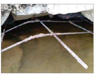
$\underbrace{\frac{\text{s}}{\text{0077}}}_{\text{NOTO}} \underbrace{\frac{\text{REINFORCEMENT EXPOSED AND CORRODED}}{\text{UNDER WEIR APRON}}$
