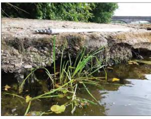
$\underbrace{ \frac{\text{B}}{\text{0074}}}_{\text{DOINTS IN MASONRY WEIR WALLS}} \underbrace{ \text{MORTAR AND FINES WASHED OUT OF} }_{\text{DOINTS IN MASONRY WEIR WALLS}}$
