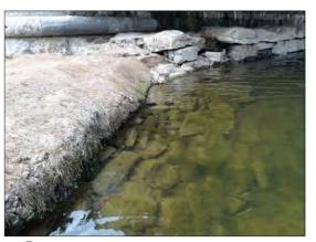
N MORTAR AND FINES WASHED OUT OF MASONRY WEIR WALL ADJACENT TO FERMOY BRIDGE
