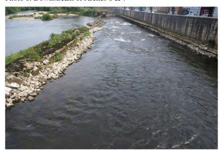
Photo 9: Flow from break in weir to left-hand side of river channel
