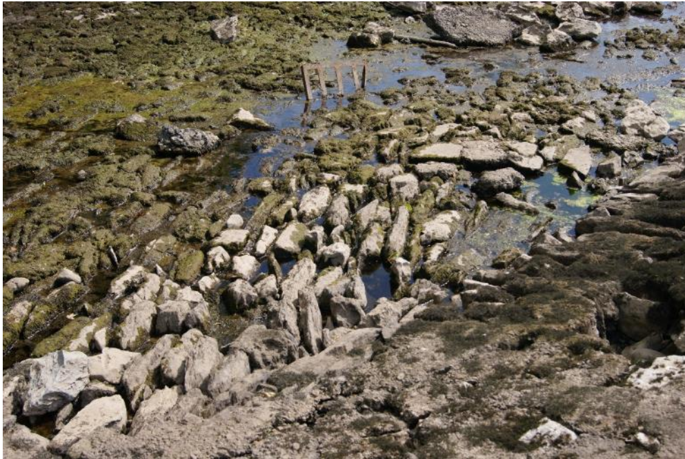
Photograph 11: Crump Weir on downstream slope with Limestone blocks clearly visible in random pattern
