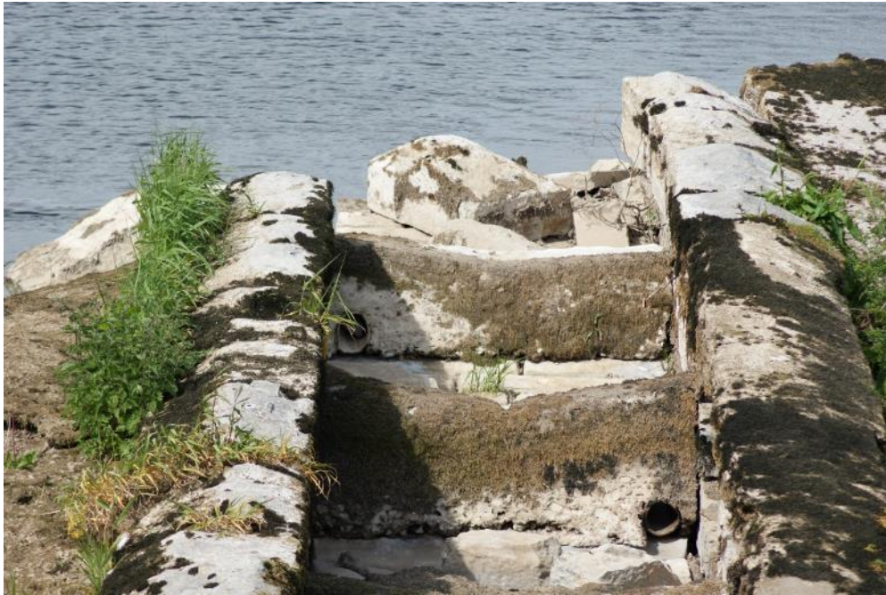
Photograph 19: Dislodged cut Limestone to Fish Pass structure
