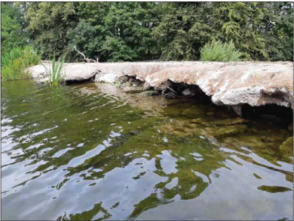
L 0076 PART OF WEIR WALL WASHED AWAY UNDER WEIR CREST
