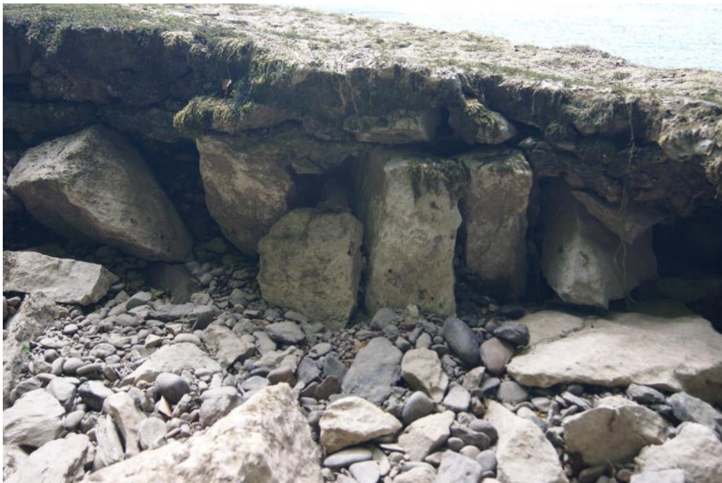
Photograph 10: Crump Weir section with concrete apron over Limestone blocks laid sideways up
