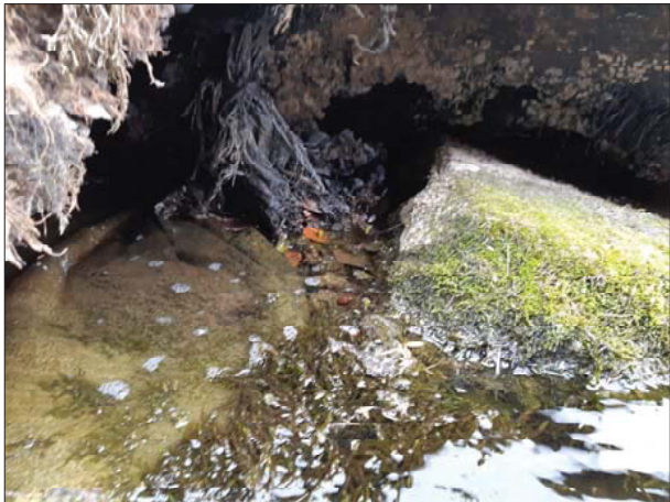
R LARGE VOIDS UNDER CONCRETE WEIR APRON
