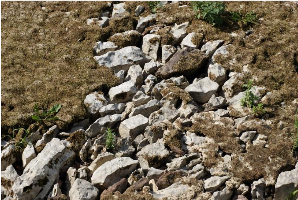
Photograph 9: Crump weir limestone of random sizes laid perpendicularly
