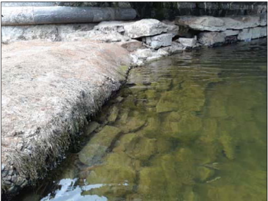
N 0076 MORTAR AND FINES WASHED OUT OF MASONRY WEIR WALL ADJACENT TO FERMOY BRIDGE
