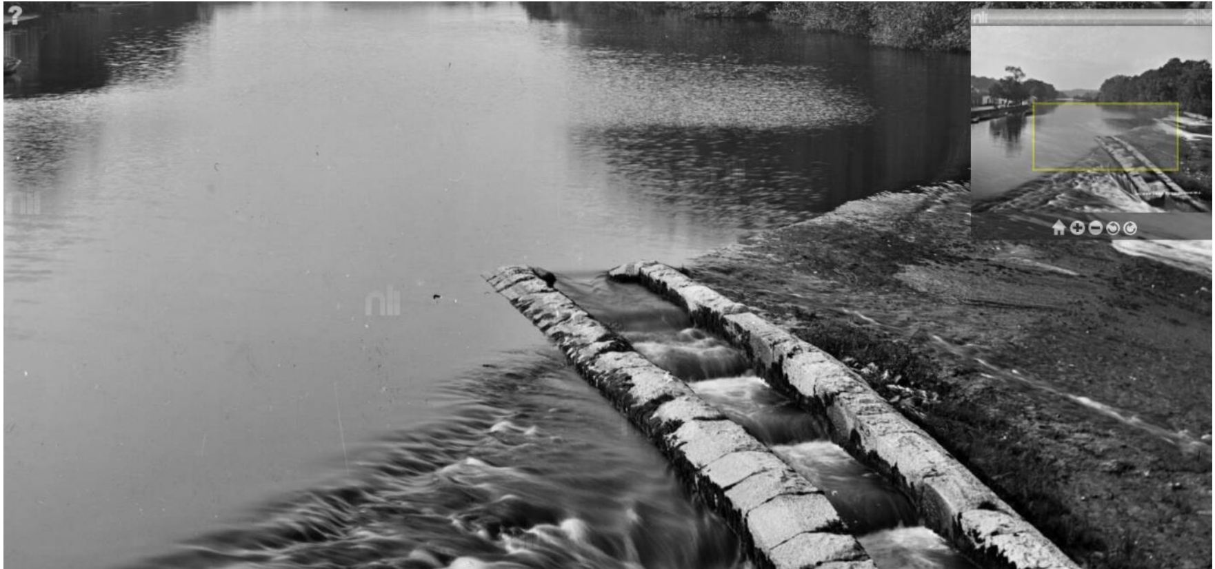
Enlargement of Above showing weir crest close to top of masonry blockwork at Fish Pass
