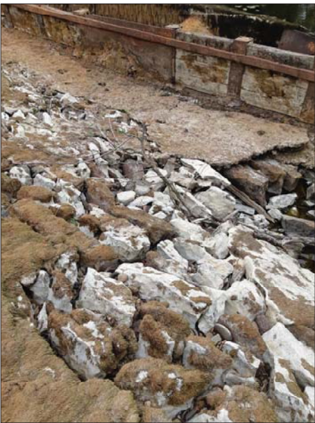
K 0076 WEIR APRON DISINTEGRATED AND WASHED AWAY AT JUNCTION WITH FISH PASS
