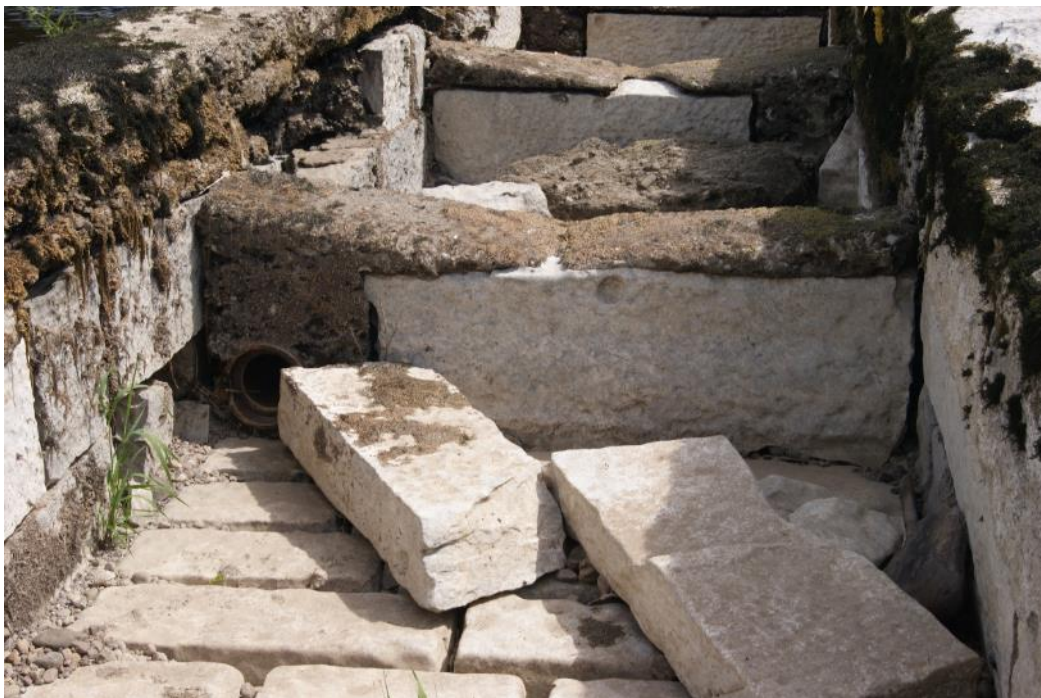
Photograph 18: Dislodged cut Limestone from Fish Pass structure
