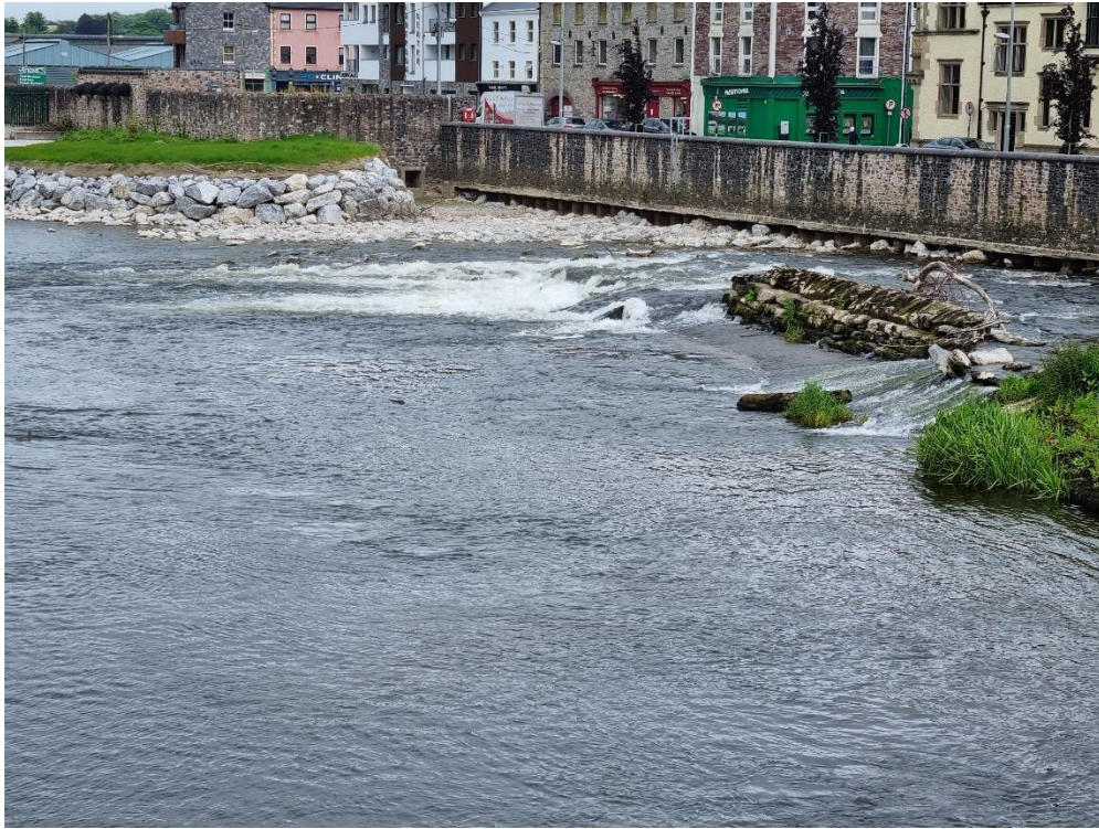
Figure 1-3: Mill Race Section of Weir & Breaches – June 2021 (Looking Downstream)
