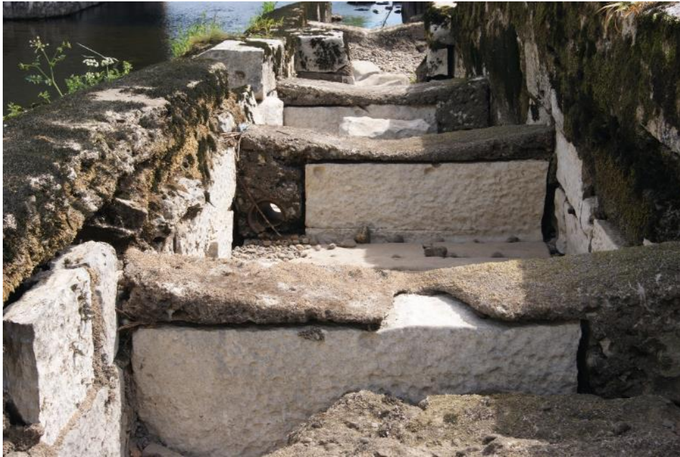
Photograph 15: Concrete capping and pipe to side intervention work within Fish Pass structure
