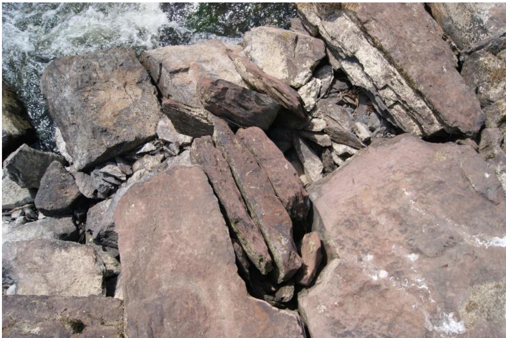
Photograph 4: Red Sandstone course on Mill Race Weir section
