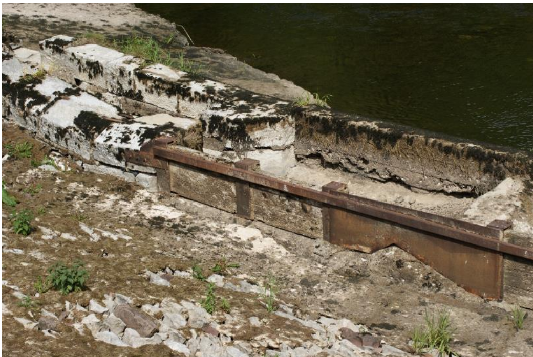
Photograph 16: Steel and timber intervention works to collapsed section of Fish Pass structure
