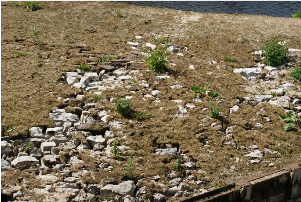
Photograph 7: View of part of back slope to Crump Weir section showing spalled concrete apron exposing original Limestone blockwork under
