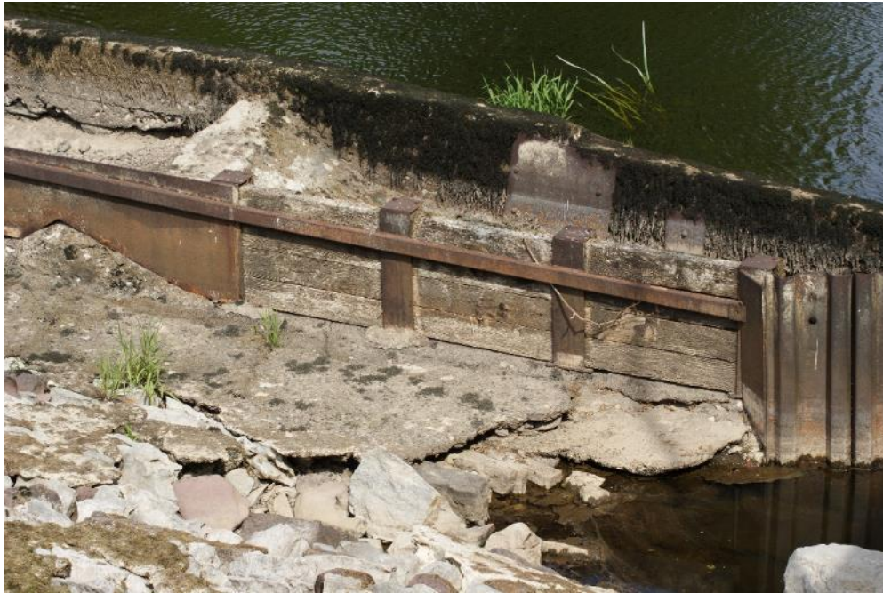
Photograph 17: Steel and timber intervention work to Fish Pass structure
