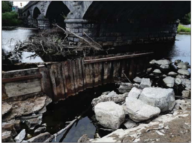
H 0075 VIEW OF TEMPORARY REPAIRS TO FISH PASS AND DISLODGED MATERIAL FROM WEIR
