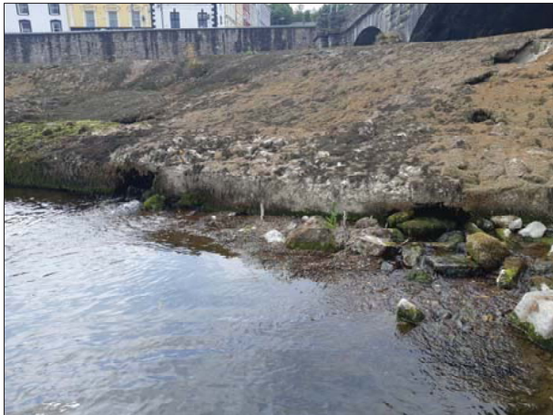
Q SURFACE OF CONCRETE WEIR APRON HAS DISINTEGRATED IN PLACES
