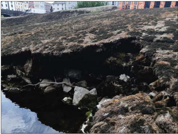
C 0074 LARGE VOID AT THE BASE OF THE DOWNSTREAM WEIR APRON
