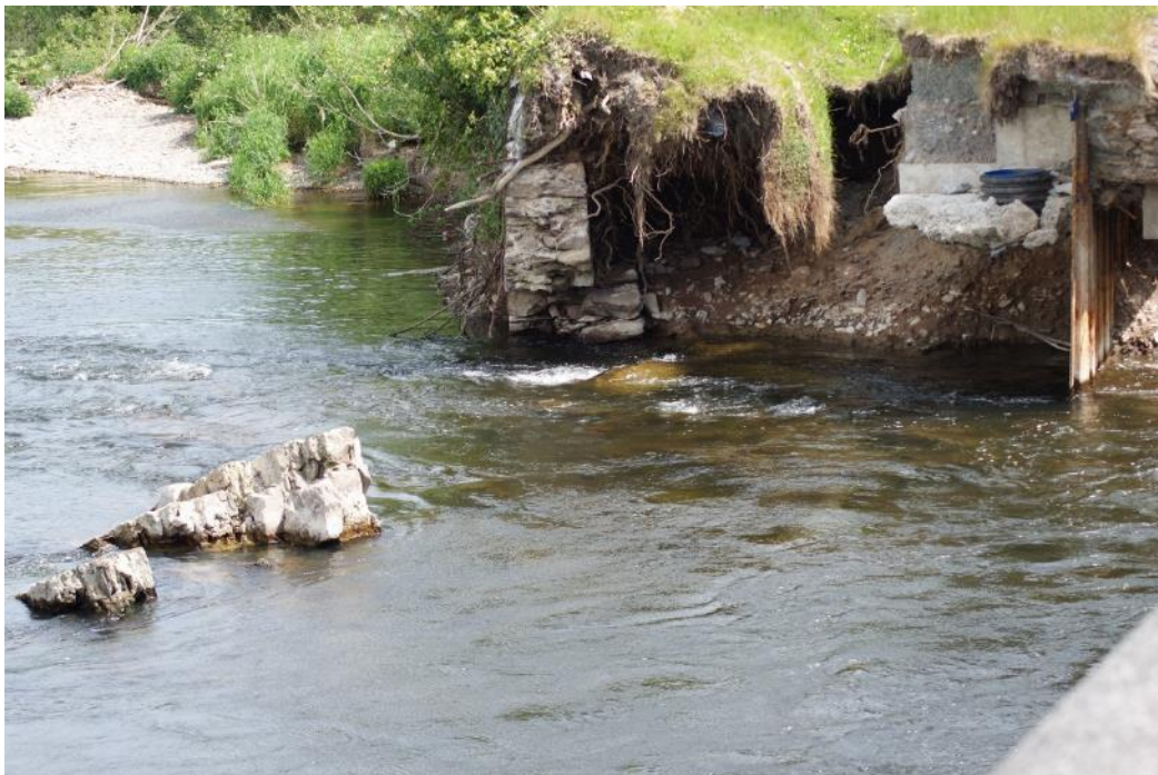
Photograph 6: Breach in weir and damage behind flood defence works
