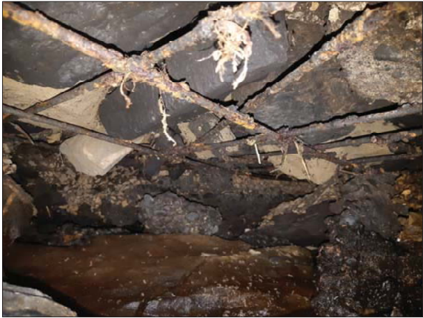
T LARGE VOIDS UNDER CONCRETE WEIR APRON, REINFORCEMENT EXPOSED AND CORRODED
