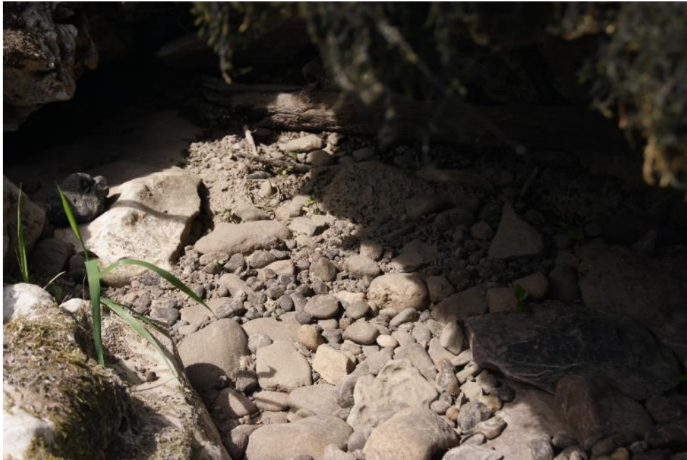
Photograph 5: Fill material within Mill Race Weir made up of random smaller stones as well as gravel
