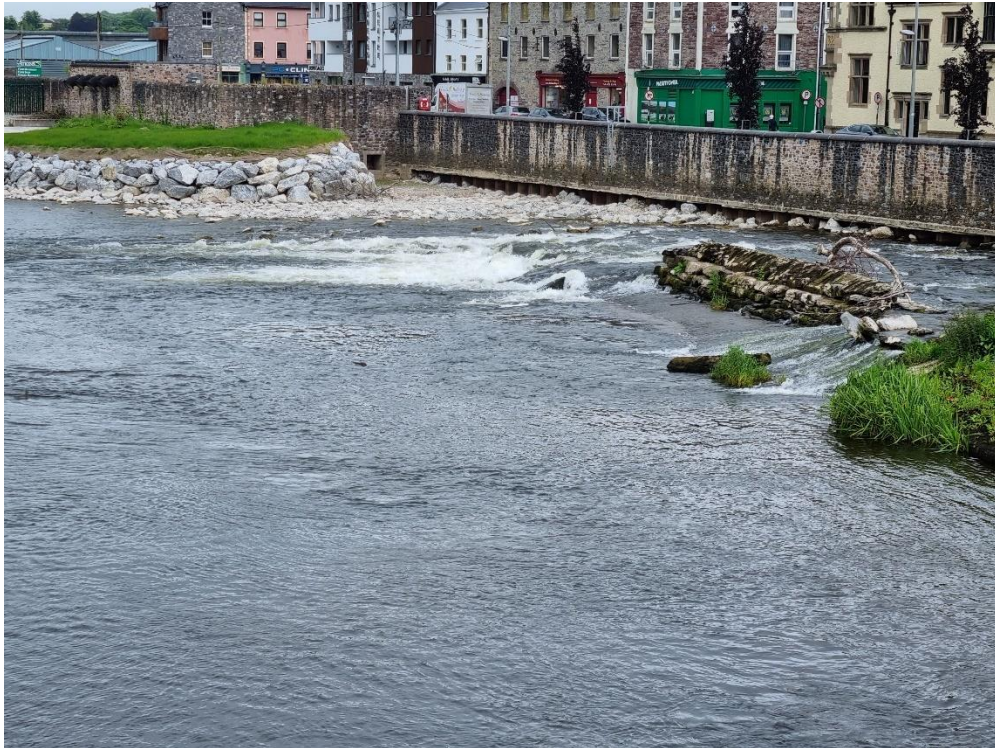
Figure 3-1: Mill Race Section of Weir & Breaches – June 2021 (Looking Downstream)
