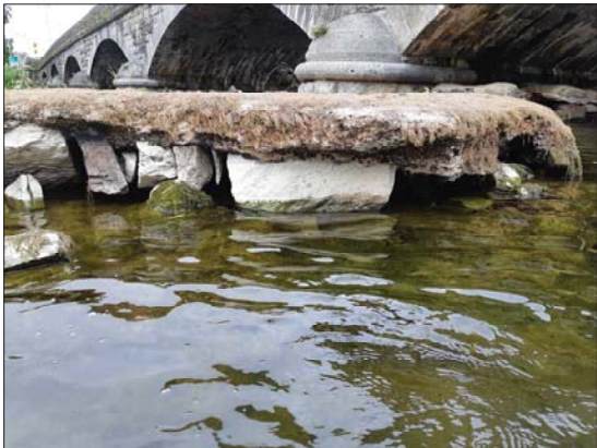
M 0076 PART OF WEIR WALL WASHED AWAY UNDER WEIR CREST
