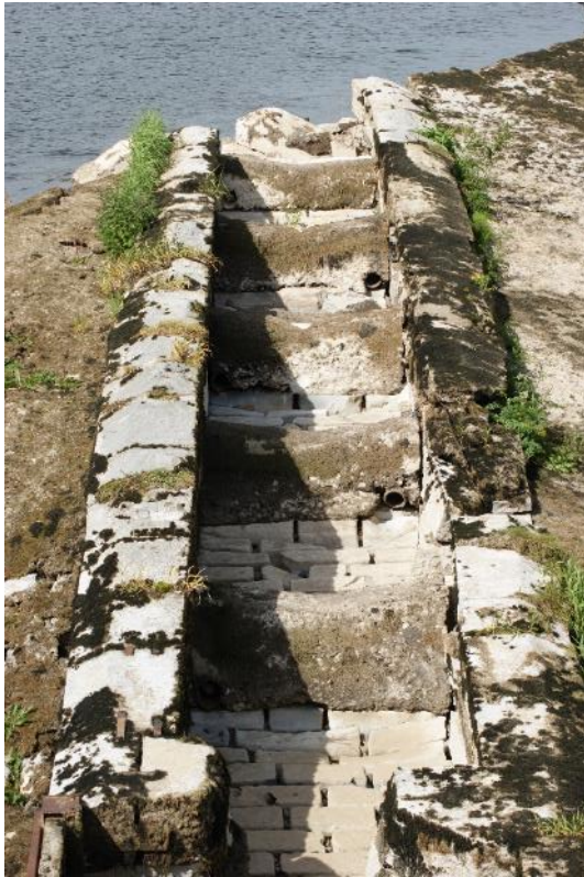
Photograph 13: Fish Pass cut Limestone construction
