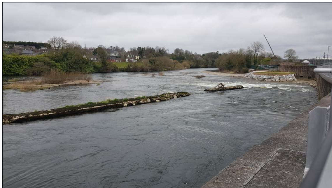
PHOTO 4 - EXISTING BREACHES IN MILL RACE SECTION OF WEIR (LOOKING DOWNSTREAM)
