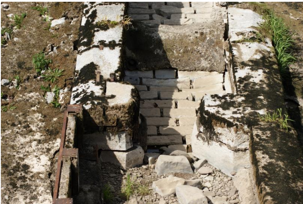
Photograph 14: Cut Limestone block construction of Fish Pass
