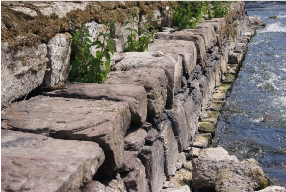
Photograph 3: Mill Race Weir section with Red Sandstone band of stonework
