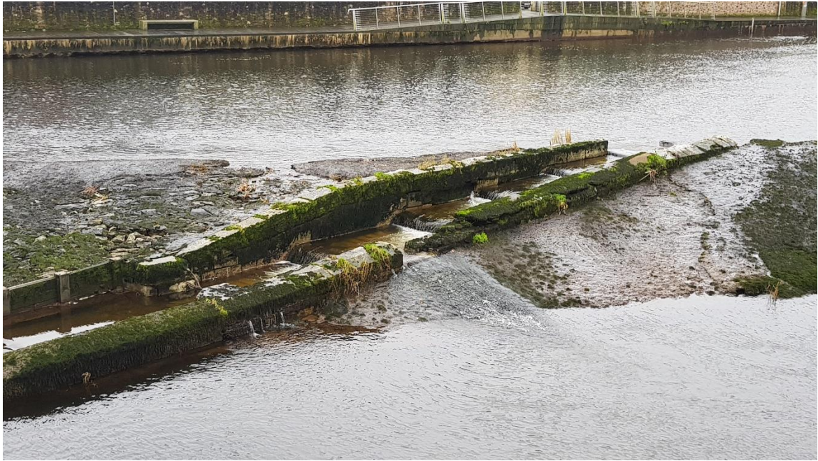
Figure 3-1: Existing Fish Pass at Fermoy Weir - November 2019
