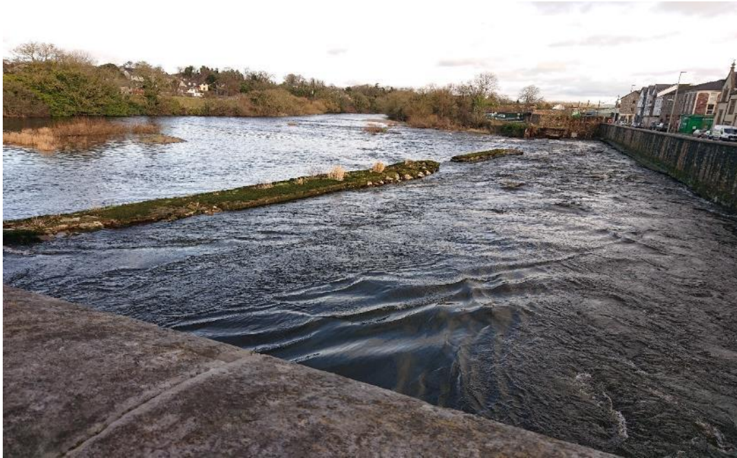
Photograph 1: View towards eastern end of weir and breached sections January 2020
