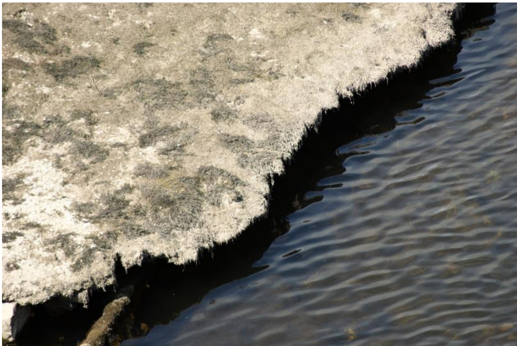
Photograph 12: Undermining of concrete apron on down slope side of Crump Weir
