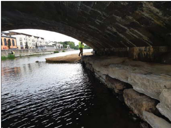
P 0076 MORTAR AND FINES WASHED OUT OF MASONRY WEIR WALL ADJACENT TO FERMOY BRIDGE
