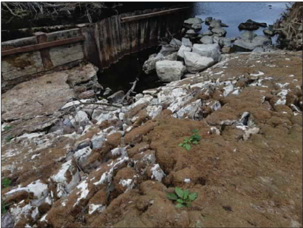
J 0076 WEIR APRON DISINTEGRATED AND WASHED AWAY AT JUNCTION WITH FISH PASS
