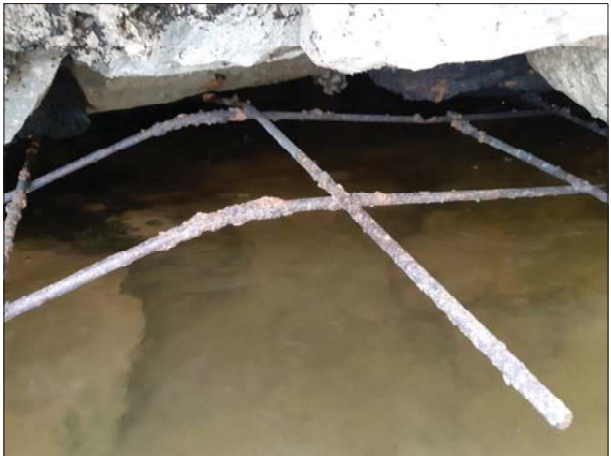
S REINFORCEMENT EXPOSED AND CORRODED UNDER WEIR APRON
