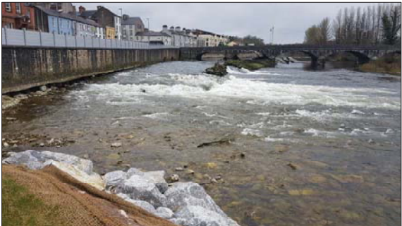
PHOTO 6 - EXISTING BREACHES IN MILL RACE SECTION OF WEIR (LOOKING UPSTREAM)
