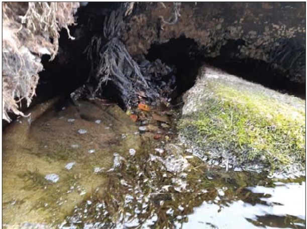
R LARGE VOIDS UNDER CONCRETE WEIR APRON
