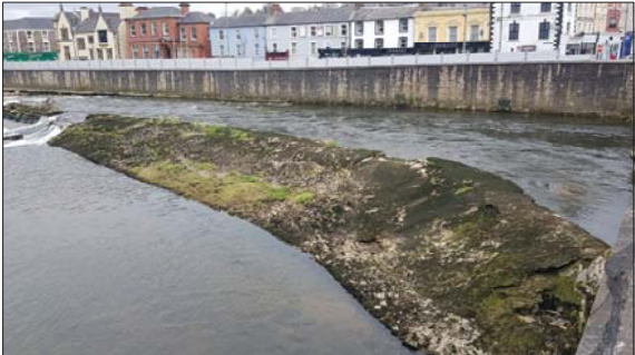
PHOTO 3 - INTERFACE BETWEEN EMBANKMENT AND MILL RACE WEIR
