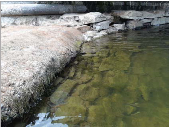
N MORTAR AND FINES WASHED OUT OF MASONRY WEIR WALL ADJACENT TO FERMOY BRIDGE
