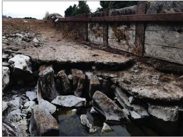
G 0075 WEIR APRON HAS DISINTEGRATED AND WASHED AWAY
