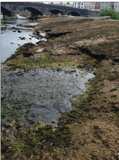
D 0074 CONCRETE APRON OF WEIR HAS DISINTEGRATED AND WASHED AWAY IN PLACES
