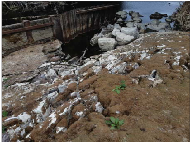
J WEIR APRON DISINTEGRATED AND WASHED AWAY AT JUNCTION WITH FISH PASS
