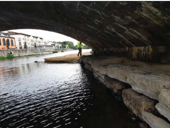
P MORTAR AND FINES WASHED OUT OF MASONRY WEIR WALL ADJACENT TO FERMOY BRIDGE
