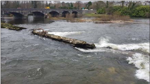
PHOTO 5 - EXISTING BREACHES IN MILL RACE SECTION OF WEIR
