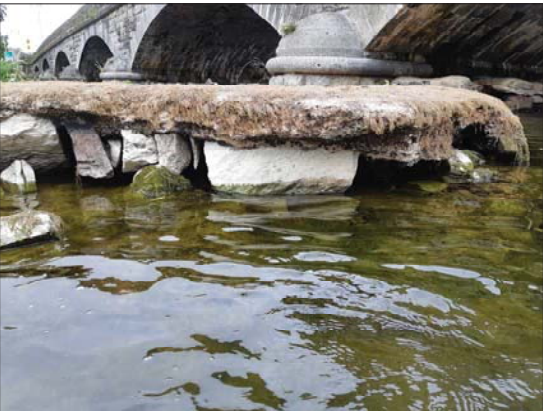
M PART OF WEIR WALL WASHED AWAY UNDER WEIR CREST
