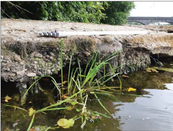
B 0074 MORTAR AND FINES WASHED OUT OF JOINTS IN MASONRY WEIR WALLS
