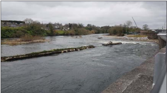
PHOTO 4 - EXISTING BREACHES IN MILL RACE SECTION OF WEIR (LOOKING DOWNSTREAM)
