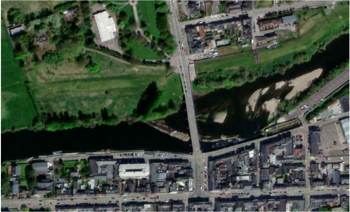
Figure 2-1: Location of site at Fermoy Bridge
