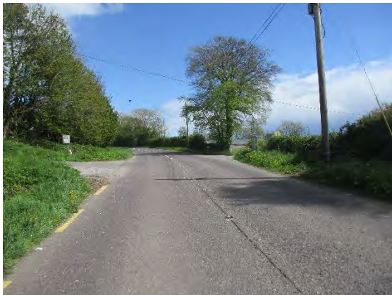
Figure 2 View at the Bowen's Cross looking North
