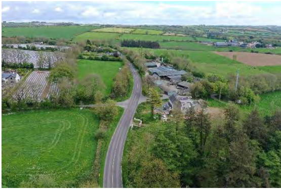
Figure 10 Aerial View at R600 Bowen's Cross looking North
