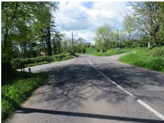
Figure 4 View looking South at the R600 Bowen's Cross
