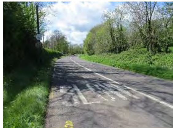
Figure 5 View looking South along R600 with Bowen's Cross at a distance
