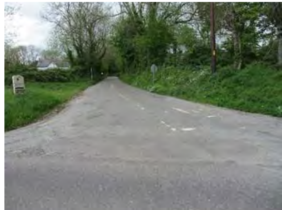
Figure 3 View looking West from Bowen's Cross into L2456 Togher Road
