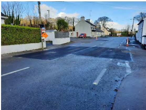
Figure 8 View looking east from the south west quadrant of the School road junction
