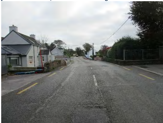
Figure 14 view looking east at the bridge
