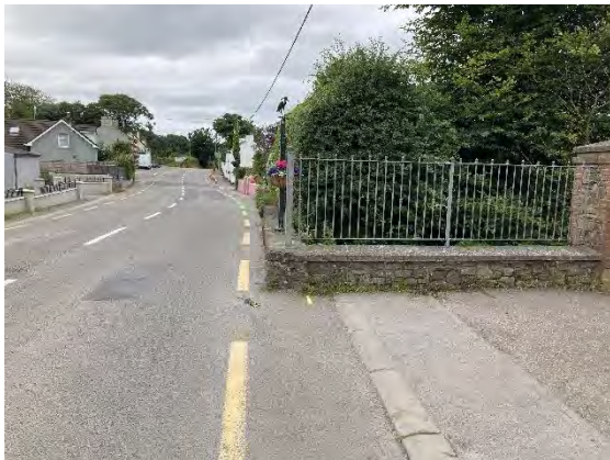
Figure 6 View looking east from before the bridge along R613 south edge
