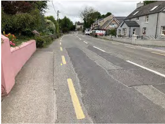
Figure 4 View looking west from before the bridge along R613 south edge with junction of L2457 and Church at a distance
