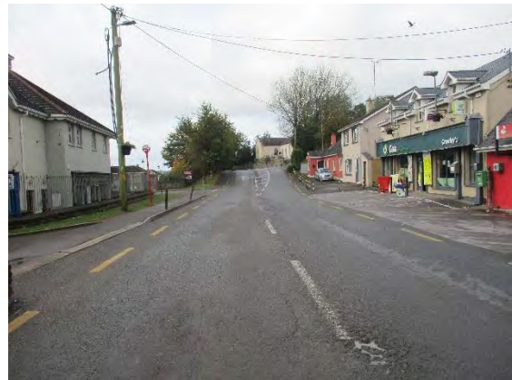
Figure 13 View looking west at the bus stops area
