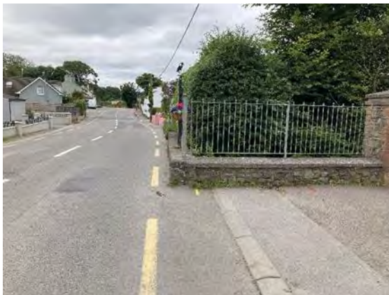
Figure 4 View looking east on the bridge
