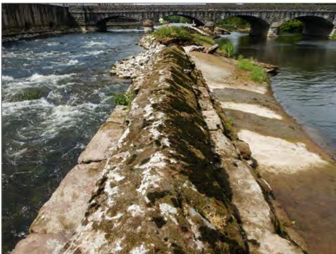
Plate 20 View from top of western end of weir, showing shaped concrete coping set back from stone courses. Taken from east.
