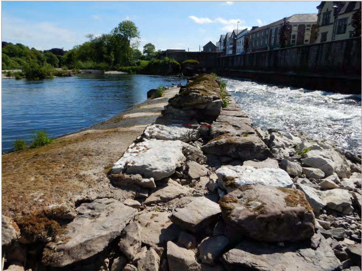
Plate 22 Random rubble fill visible at small breach. Taken from east.
