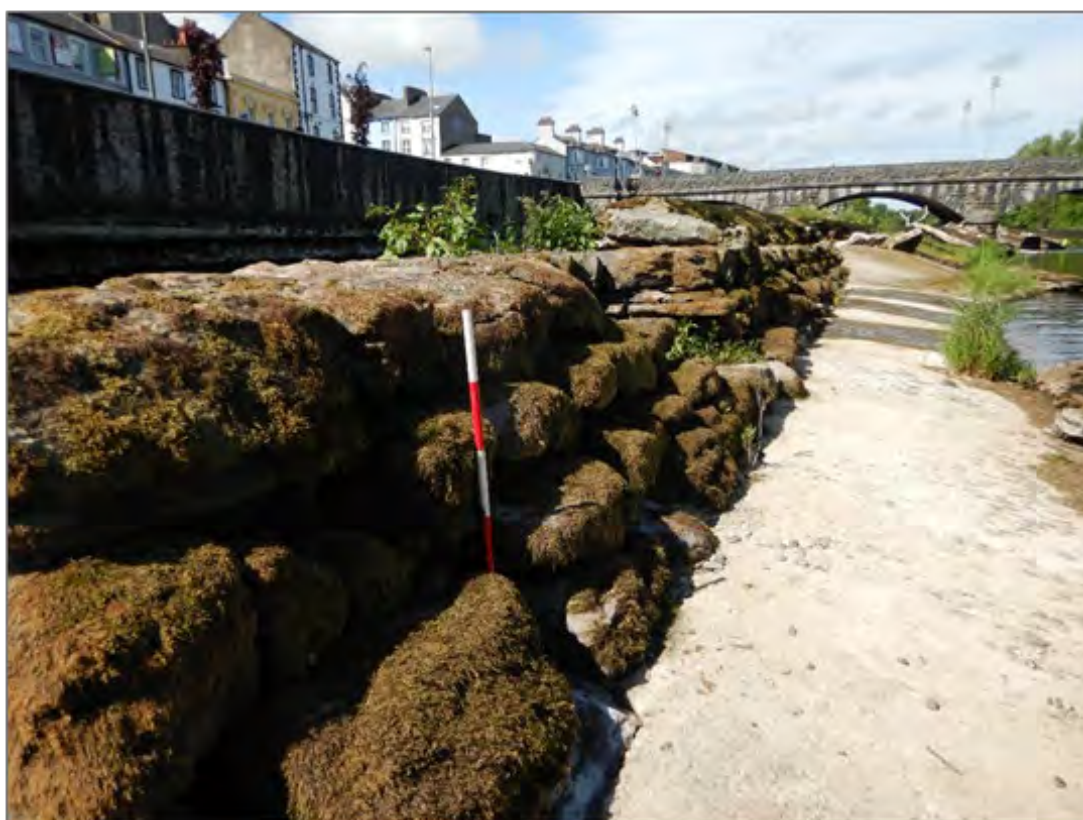
Plate 21 Stepped courses of stone on north face of western end of weir. Taken from west.
