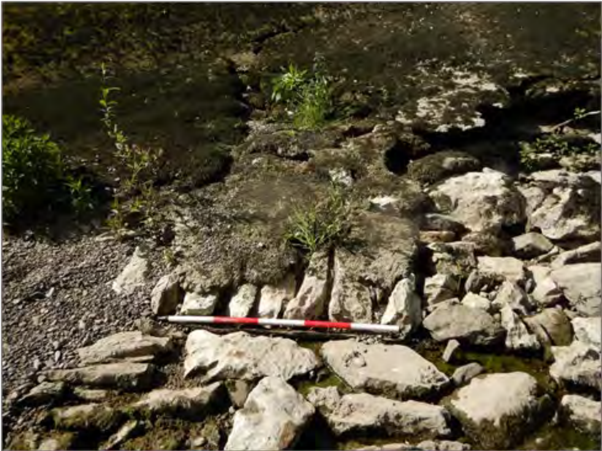
Plate 15 Timber separating end of weir and paving stones, taken from north-east.
