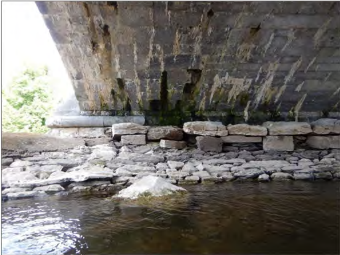
Plate 16 Original rubble stone slope of weir capped by two courses of large cut limestone, ending at the end of the pier of Fermoy Bridge. Taken from south.
