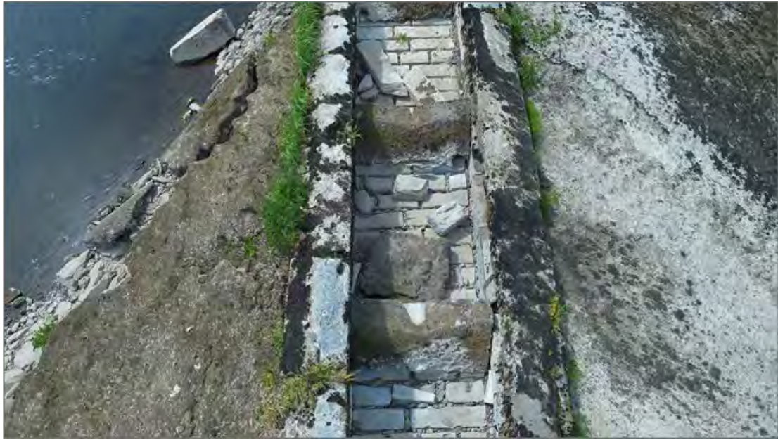
Plate 23 Aerial of fish pass, showing paving stones at the base.
