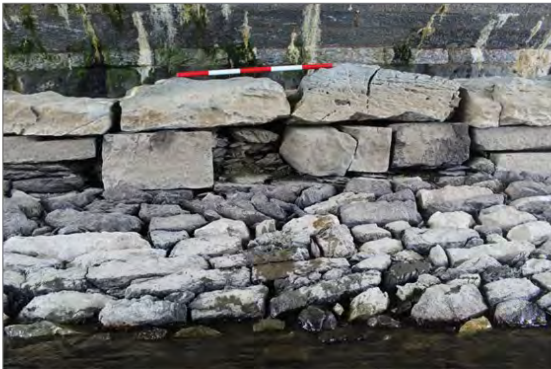
Plate 17 Original rubble limestone slope with two/three courses of large limestone cut stones overtop. Taken from south.
