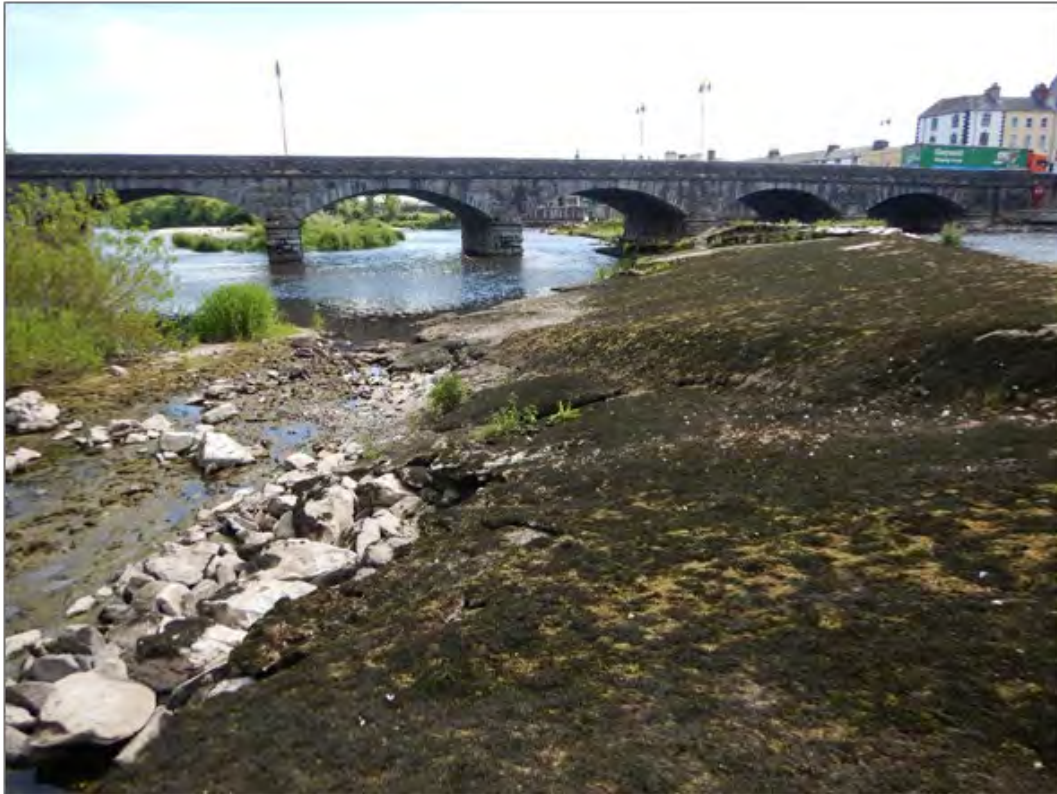
Plate 9 Concrete-covered slope of fish pass east of the bridge, showing paved stone area to the left. Taken from north-east.
