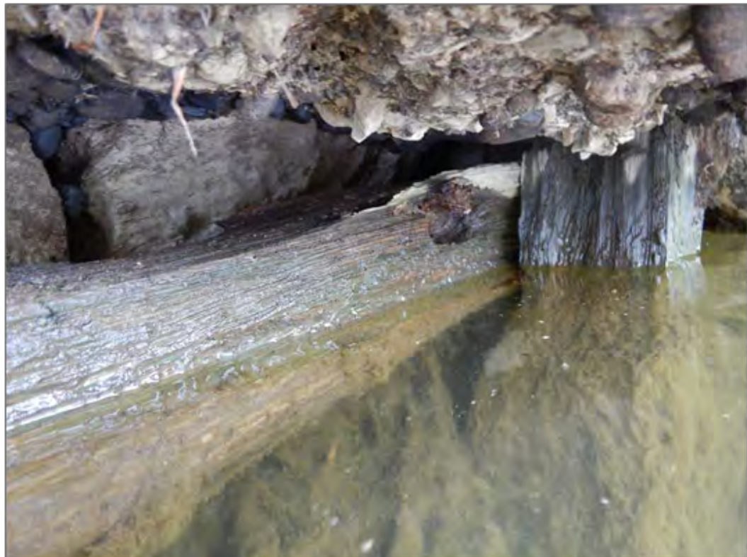
Plate 12 Timber baulk underneath concrete of weir slope, with stones visible behind (left) of the timber and upright timber (right). Taken from east.
