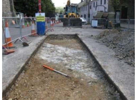
Plate 50: Sub-surface town wall foundation base (Emmet Row – Tobar Archaeological Services).
