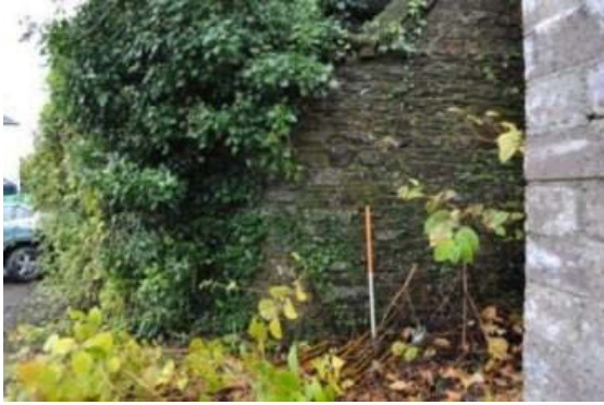
Plate 42: Rounded north-east corner of wall, looking south.
