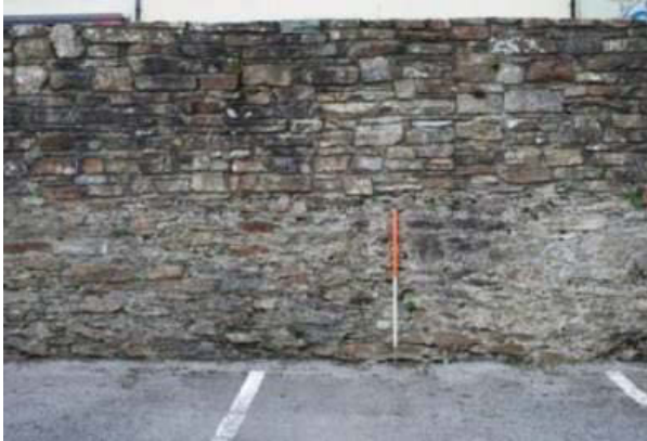
Plate 6: East (internal) elevation of original town wall beneath modern rebuild.
