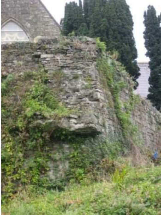
Plate 66: Plantlife to southeast corner. Note potential flanker to corner
