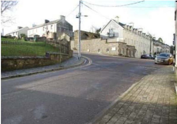
Plate 94: Site of West Gate at O'Mahony Ave./Ballymodan Place.
