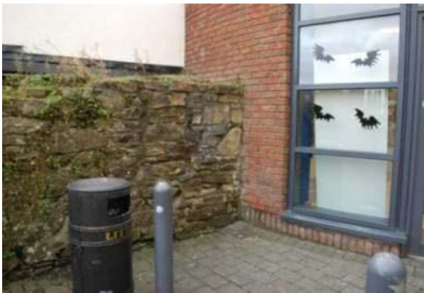
Plate 10: West elevation of wall where it adjoins shopping centre building.
