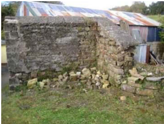
Plate 91: Concrete render to potential structure
