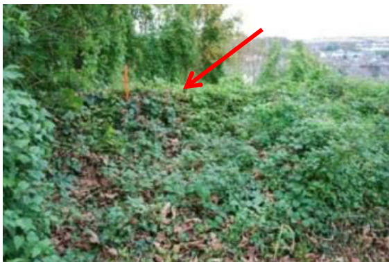
Plate 27: Overgrown wall on line of town wall, Section 9 west of church steps.
