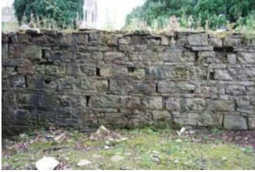
Plate 45: Later construction method in north elevation of Section 14.
