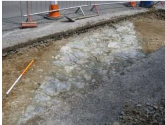
Plate 104: Stone feature F1, Emmet Row, possible foundation of town wall.
