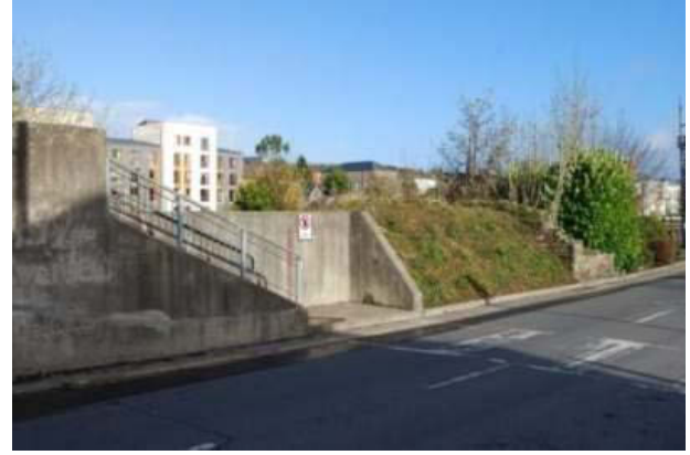
Plate 4: Concrete steps and metal railings to west of Section 1, looking north-east.
