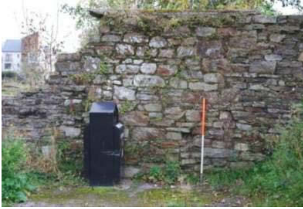
Plate 3: Detail of west elevation, Section 1.
