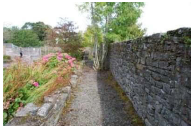
Plate 13: Central core of wall (Section 2), looking north-east.
