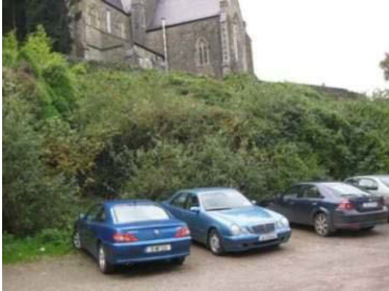
Plate 70: East-facing elevation of wall which could not be surveyed.
