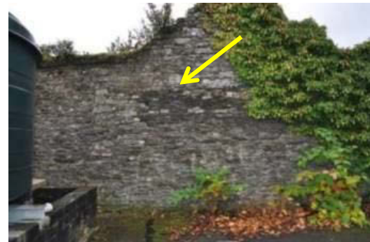
Plate 41: East elevation of Section 13 from P.O. yard. Note original masonry (arrow) with later rebuild on top.
