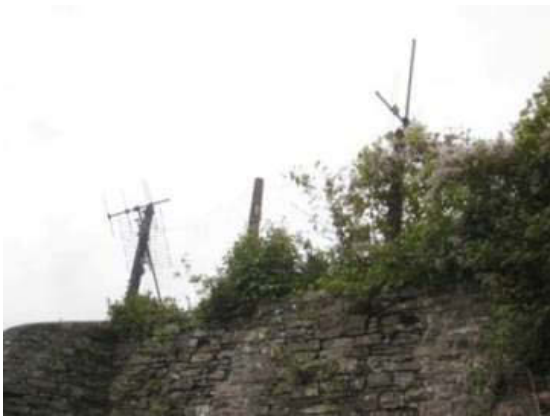
Plate 74: Post and wire fence to top of wall. Note presence of TV aerials also
