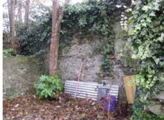
Plate 83: View of wall to rear of No. 6 from southwest
