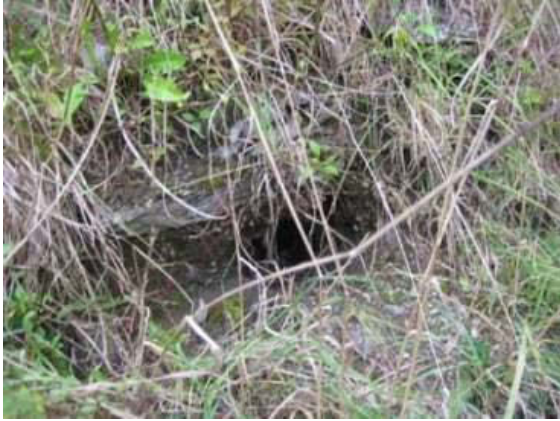
Plate 64: Animal burrowing beneath Section 4
