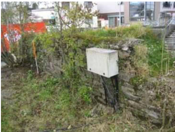
Plate 58: Fisheries Board box to east elevation of west wall.
