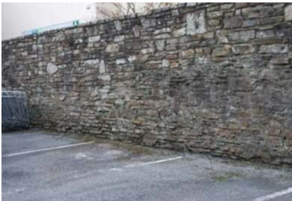
Plate 7: Original wall surviving to varying heights beneath modern rebuild (East elevation).
