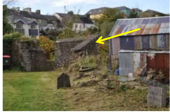
Plate 46: Possible earlier feature at west end of Section 14, looking west north-west.
