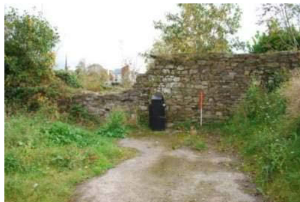
Plate 2: West (external) face of Section 1, note location of litter bin and earthen bank to right.
