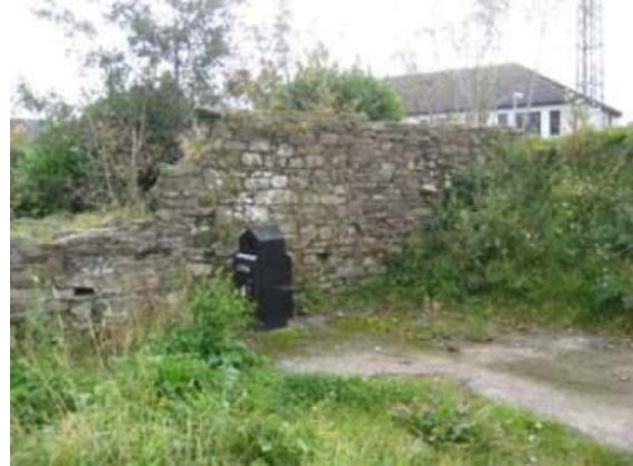
Plate 59: West elevation of west wall with litter bin
