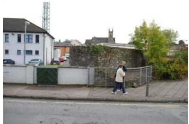
Plate 12: North-east end of Section 2, looking south.
