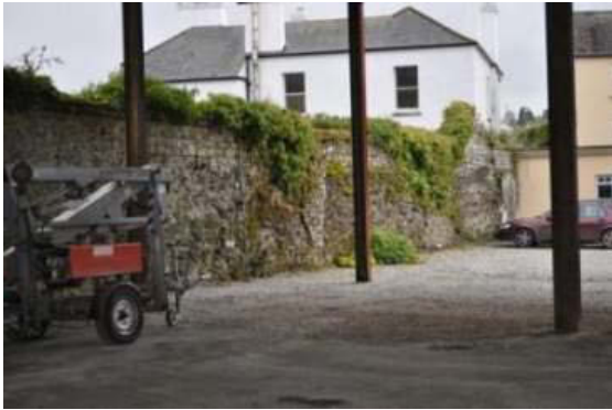
Plate 43: West elevation (Section 13), looking south-east.
