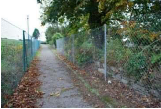
Plate 30: Link fence along line of town wall, Section 9, looking south-west.
