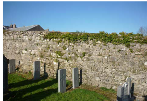
Plate 51 View along re-built wall to St. Mary's churchyard.
