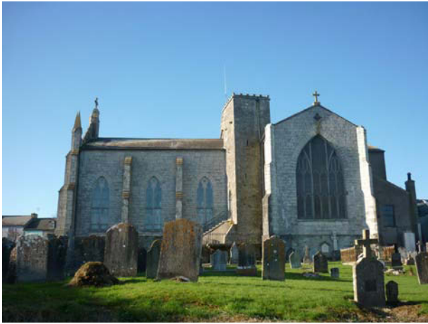
Plate 17 View of St. Mary's & Desmond's Tower from east.
