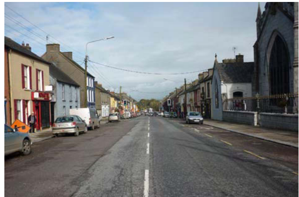
Plate 8 View looking north along Main Street.
