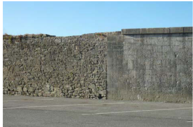
Plate 28 View of rubble wall beside ashlar wall to barracks.
