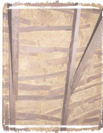
Figure 16. Detail of scraw, Lisnacore, near Kanturk, North Cork. CCC No 200.
