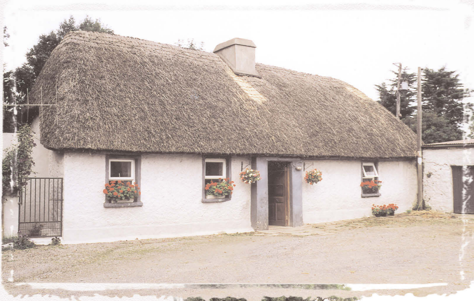
Figure 9. Example of lobby-entry thatch house, Glenabulla Cross, Mitchelstown, North Cork. CCC No 58.
