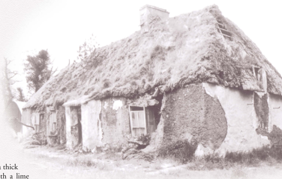
Figure 19. Exposed Clay in a ruinous thatched house, Milltown, near Charleville, North Cork. CCC No 21.
