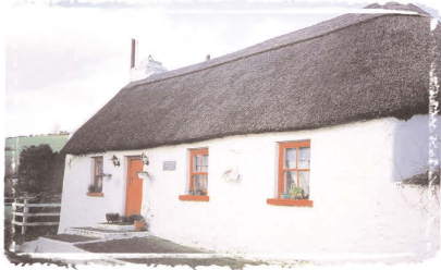
Figure 12. Example of a half-gabled thatched roof, at Knockmonalea West, Youghal, East Cork. CCC No 144.
