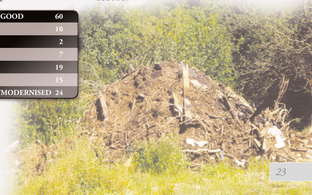
Figure 30. Disintegrated thatched house, Shandrum. CCC No 9.
