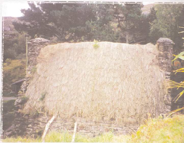
Figure 15. Ciób roof in sole remaining West Cork house, near Glengarriff, Coolieragh. CCC No 185.
