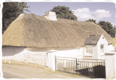
Figure 13. Example of a hipped roof, North Cork. CCC No 207.
