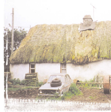
Figure 14. Wheaten straw roof, Balinure, Bartlemy, East Cork. CCC no 209.
