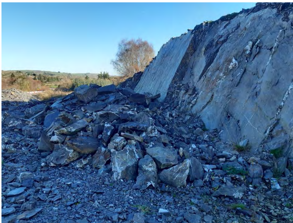
Plate 6. Cutaway rock outcrop at the south-eastern side to facilitate the road realignment
