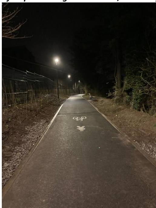
Typical cycleway lighting
