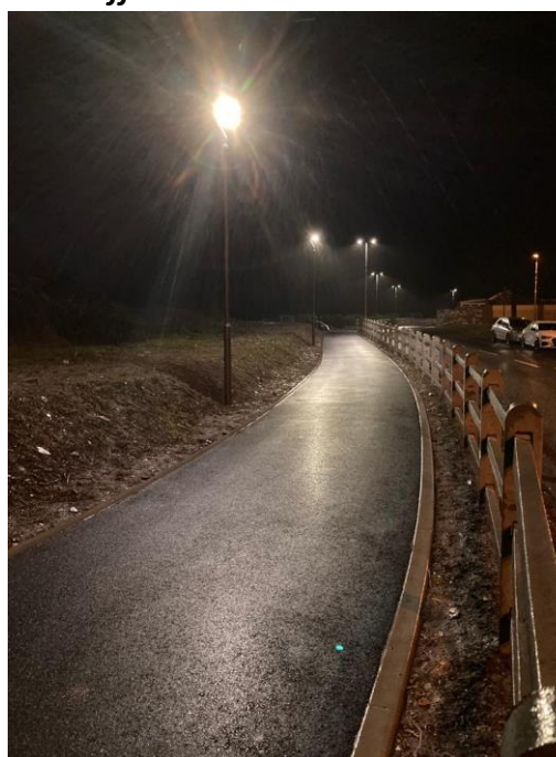
Typical walkway lighting
