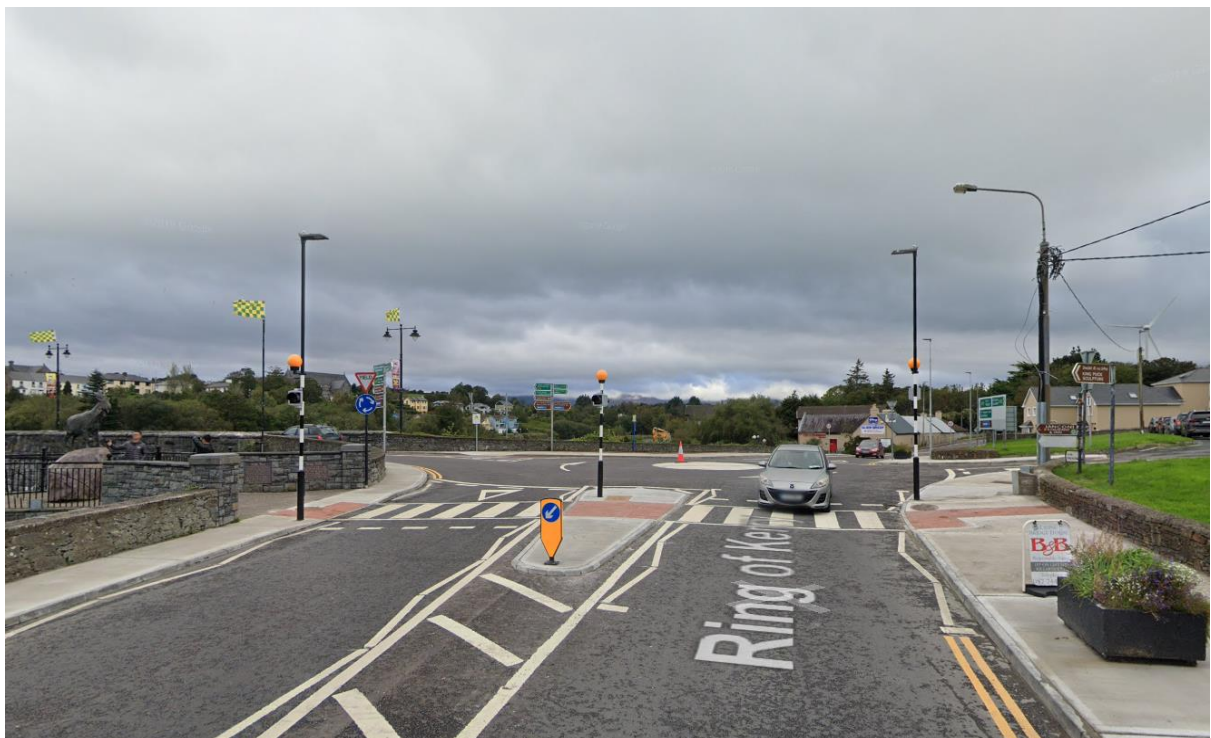
Zebra auxiliary lighting integrated into traffic signals
