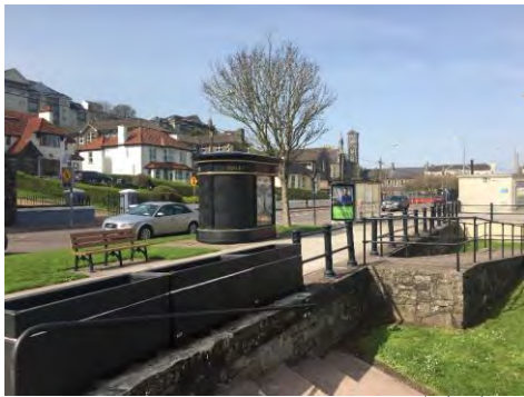
1. Service structures contained in northwest area
