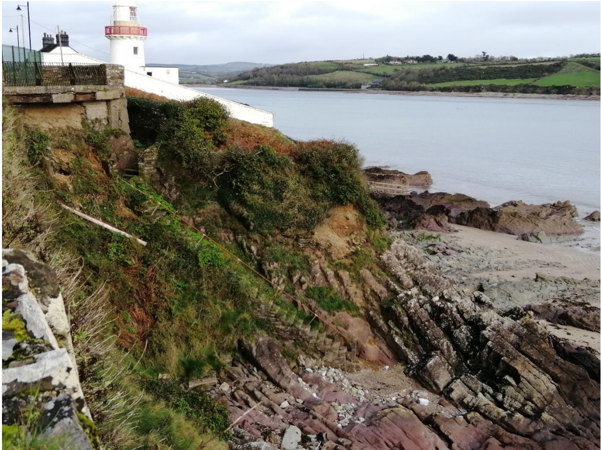
Plate 3 Photograph of existing Lighthouse Road Viewing Platform facing northeast
