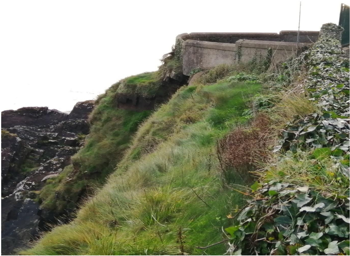
Plate 2 Photograph of existing Moll Goggins platform facing south
