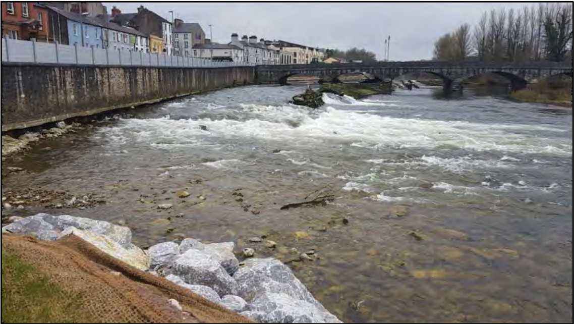
PHOTO 6 - EXISTING BREACHES IN MILL RACE SECTION OF WEIR (LOOKING UPSTREAM)
