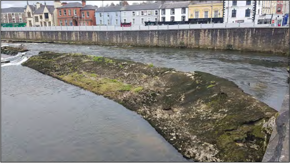
PHOTO 3 - INTERFACE BETWEEN EMBANKMENT AND MILL RACE WEIR
