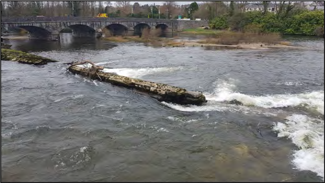
PHOTO 5 - EXISTING BREACHES IN MILL RACE SECTION OF WEIR
