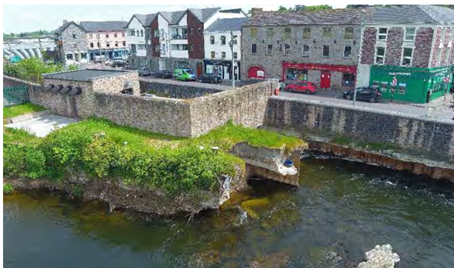
Figure 4-1: Bank Erosion at Mill Island following breach in weir
