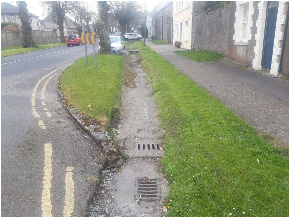
Figure 2 – Existing Open Channel Drain
