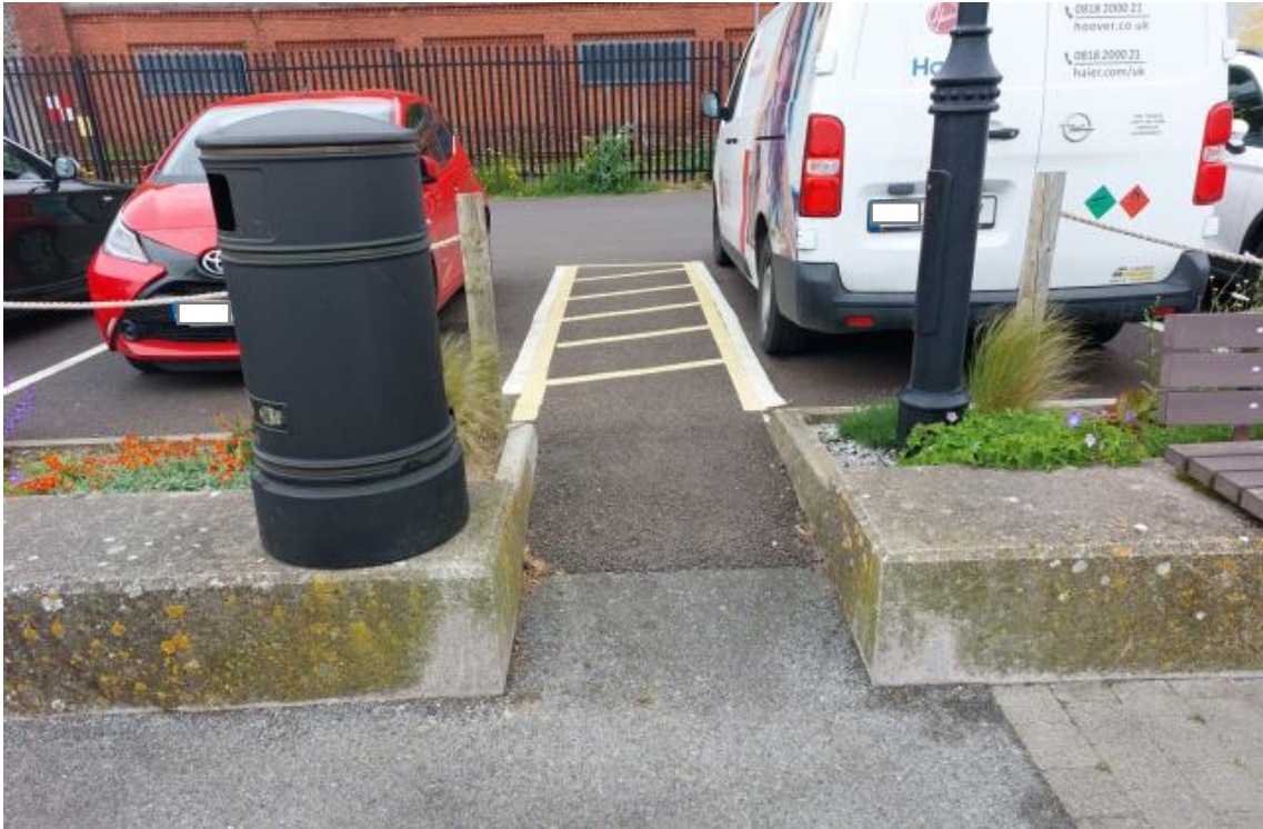
Figure 3.2: Pedestrian access through concrete wall
