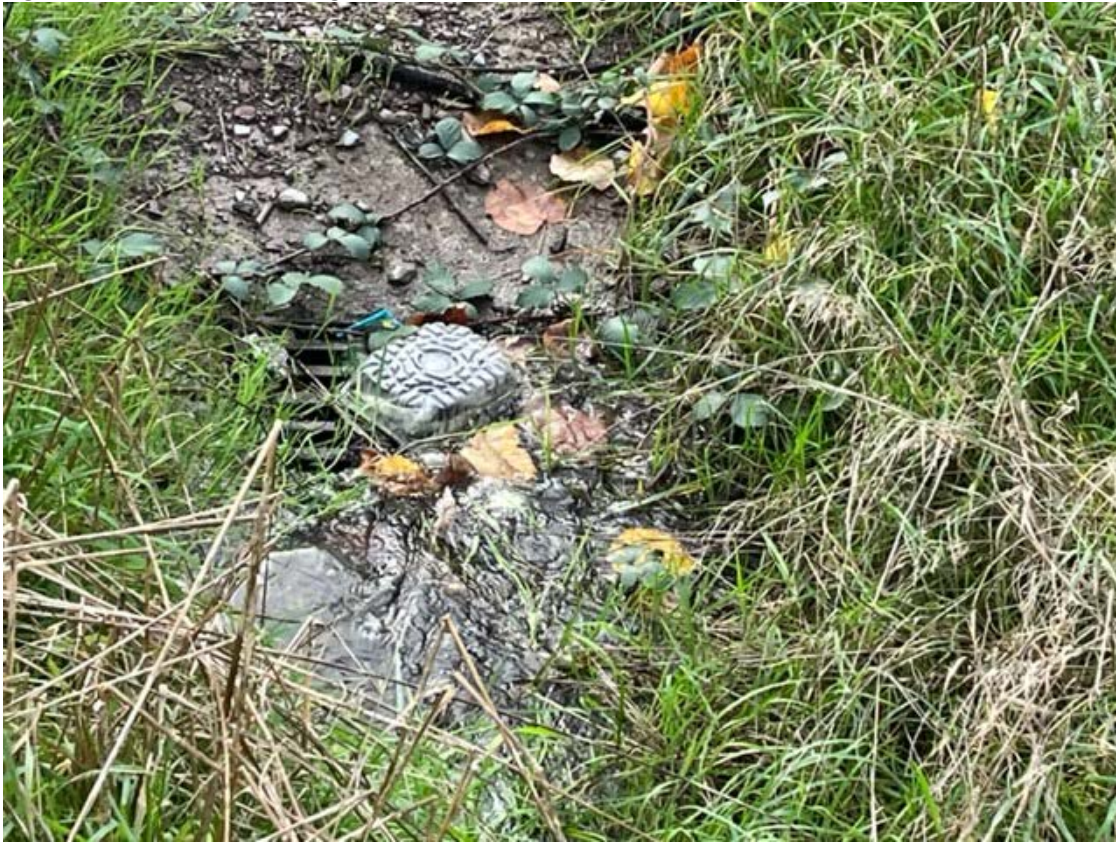
Figure 2.0: Picture indicating Watercourse entering Road Gully at Roadside
