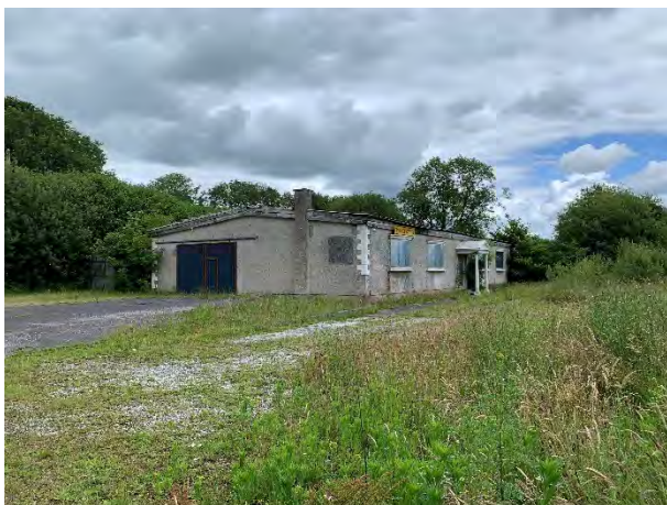
Plate 3-3: Disused commercial building within the UEA area
