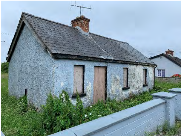
Plate 3-4: Disused house located adjacent to Cork Road
