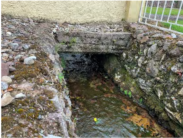
Plate 3-8: Concrete culvert under entrance to domestic property
