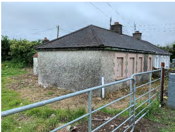
Plate 3-5: Disused house located adjacent to the bus stop at Cork Road
