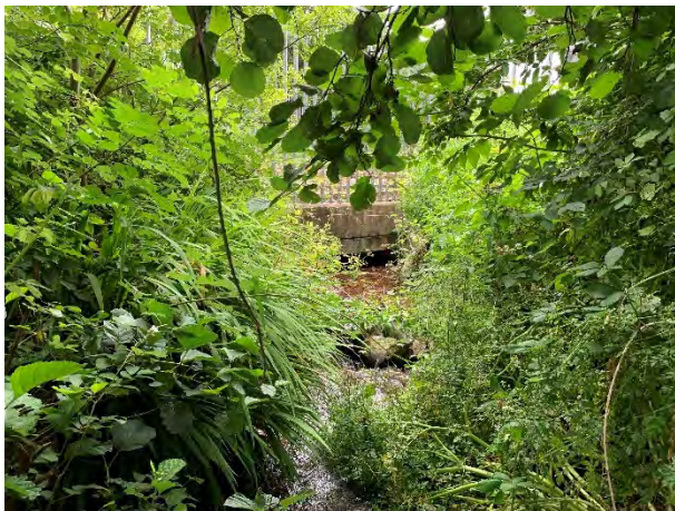
Plate 3-7: Low Lying culvert under railway line
