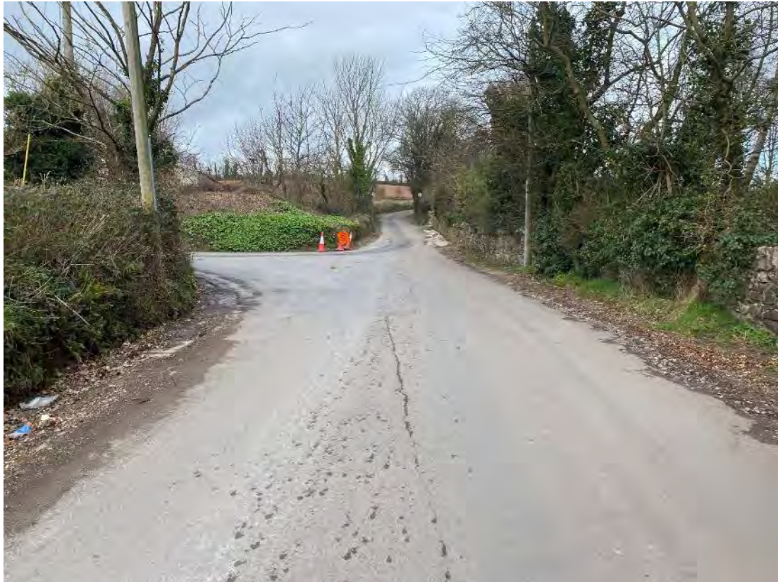
Plate 47: T-junction for upgrading to the north of Greenville house – note the demesne wall
