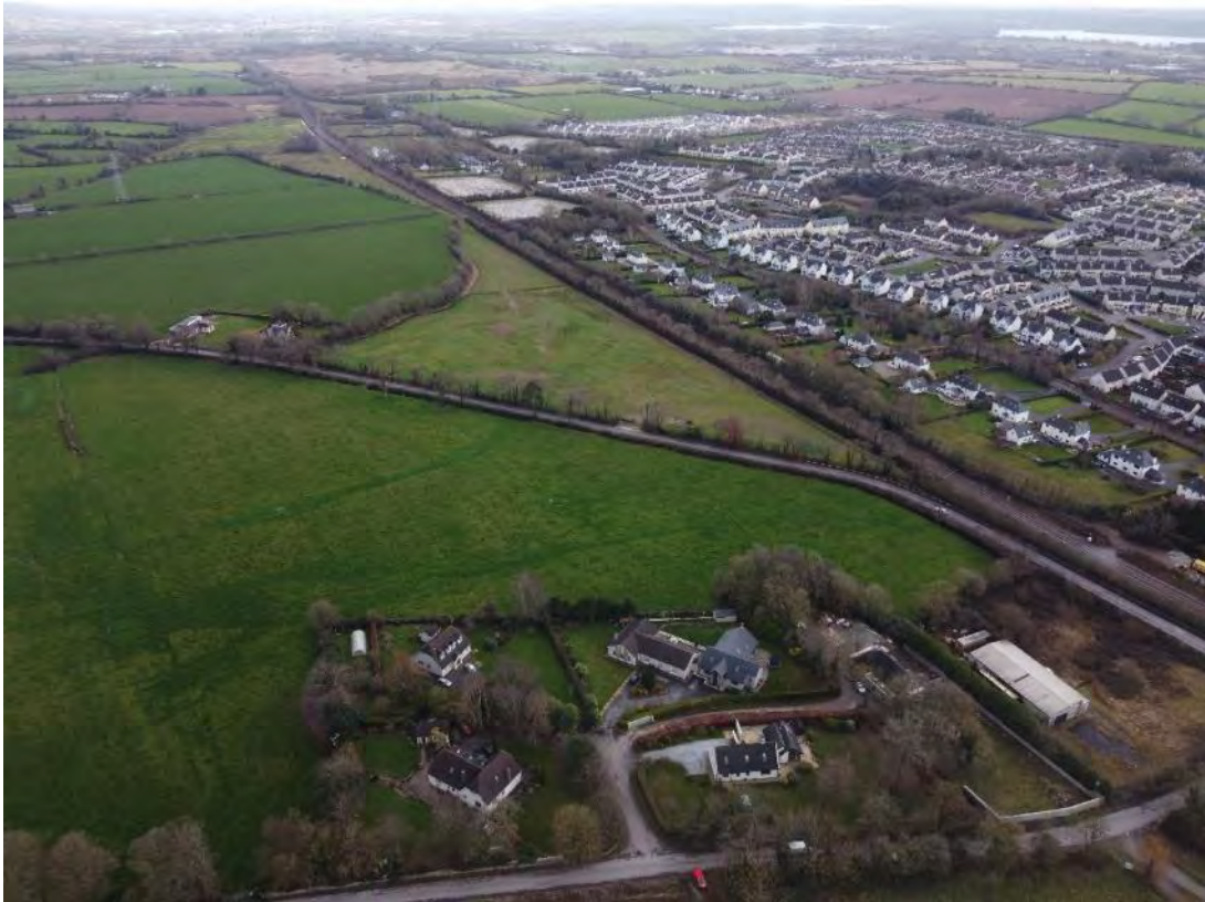
Plate 21: Drone view of Field 9, facing southwest-note warehouse to bottom right of frame due for demolition.
