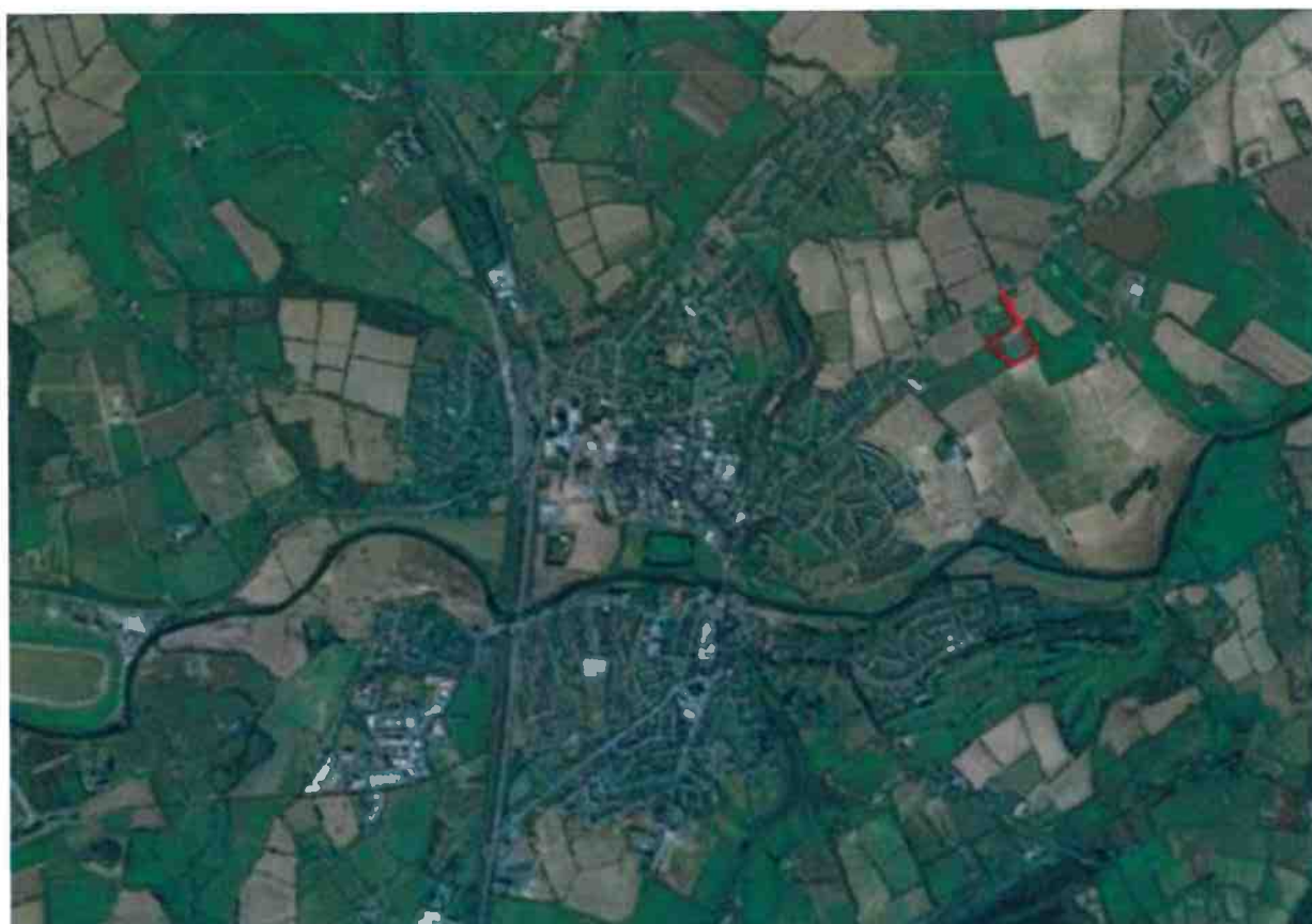
Fig 1.0 Location of Mallow 110kV Substation, outlined in red, in the context of Mallow
