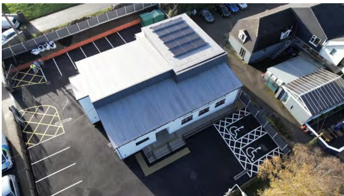
Ringaskiddy Community Hall (new roof)
