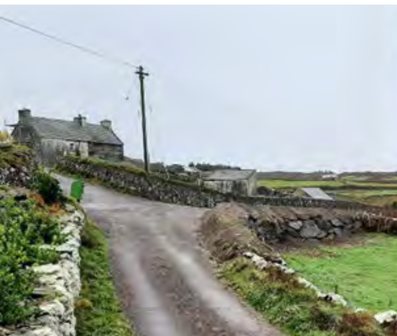
Cape Clear - new retaining wall, and roadworks
