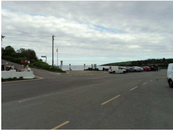
Figure 2 View from west road edge of R612 looking south towards the Fountainstown Beach
