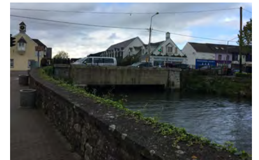
Cork Road bridge
