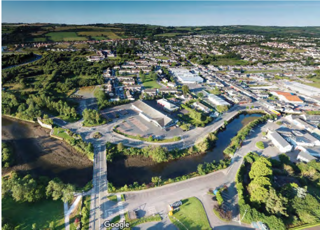
Aerial view of the site
