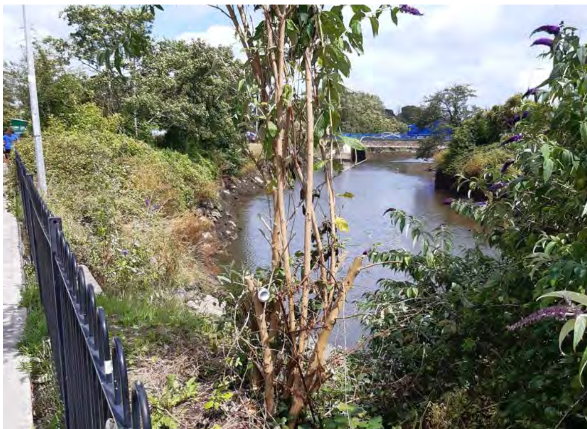
Figure 2-5 - Existing Railing and River Embankment
