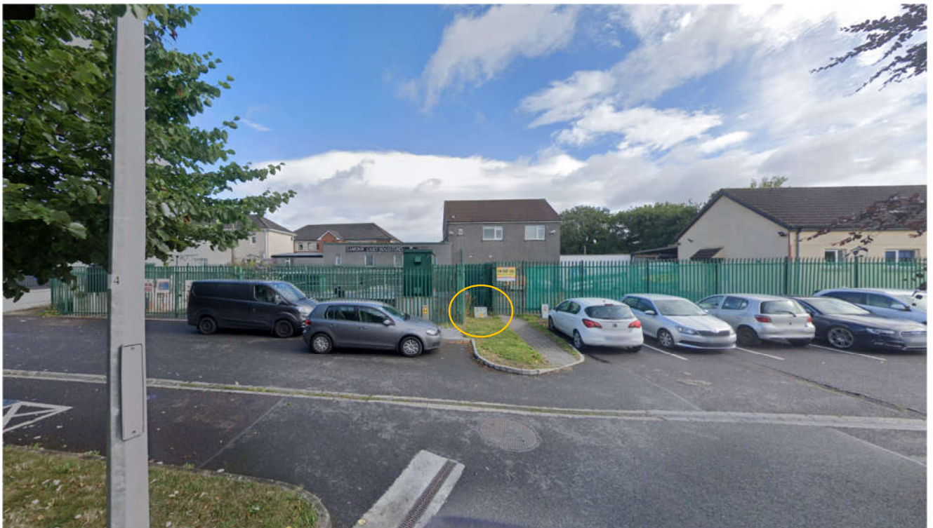
Figure 2-3 - Potentially Undergrounded ESB Cable
