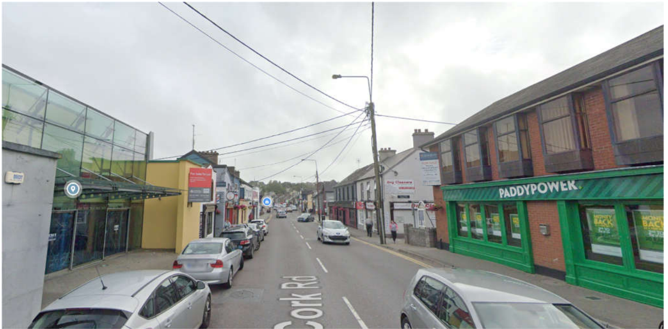
Figure 2-2 - Main Street Electricity Pole
