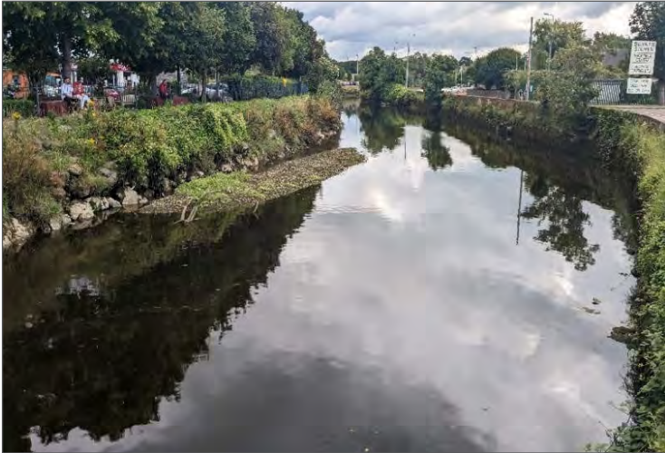
Plate 4.4 View downstream of the proposed works area from R611 bridge.
