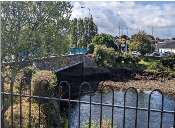
Plate 4.5 Bridge at eastern boundary of the proposed works site on which the R612 lies (TII Bridge ID: CC-R612-001.00).
