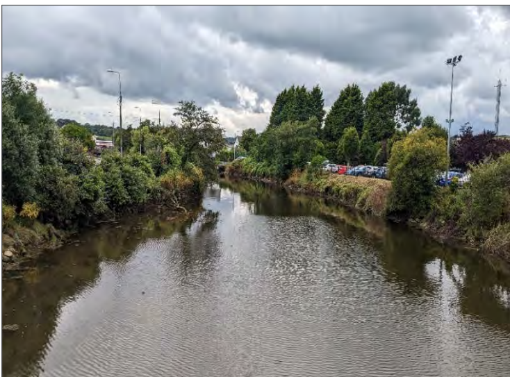
Plate 4.6 View upstream from CC-R612-001.00 of the proposed works area.
