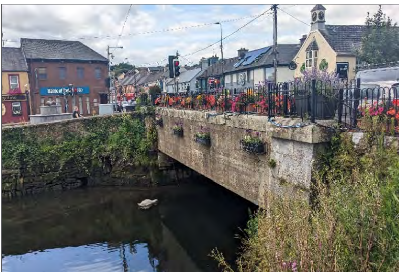
Plate 4.3 Bridge at western boundary of the proposed works site on which the R611 lies (Main Street, Carrigaline) – foraging Mute Swan present.
