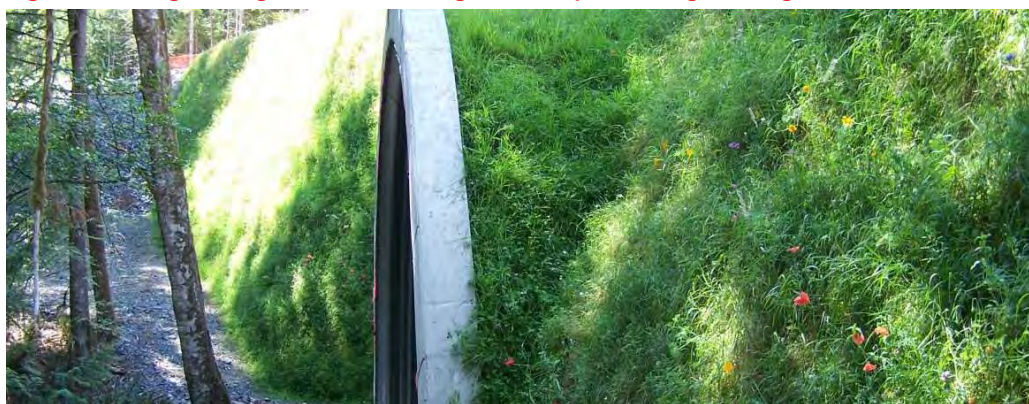
Figure 4.19: Vegetated green wall retaining solution, following vegetation growth
