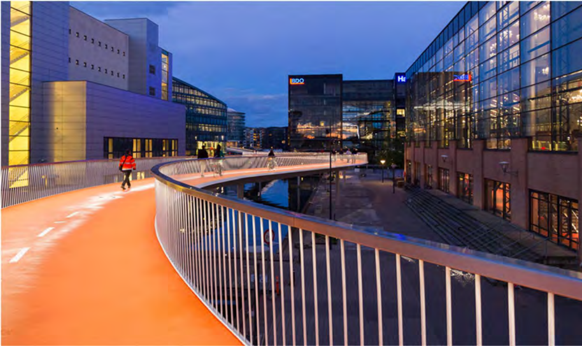
Figure 16.9: Parapet type with vertical parapet infill
