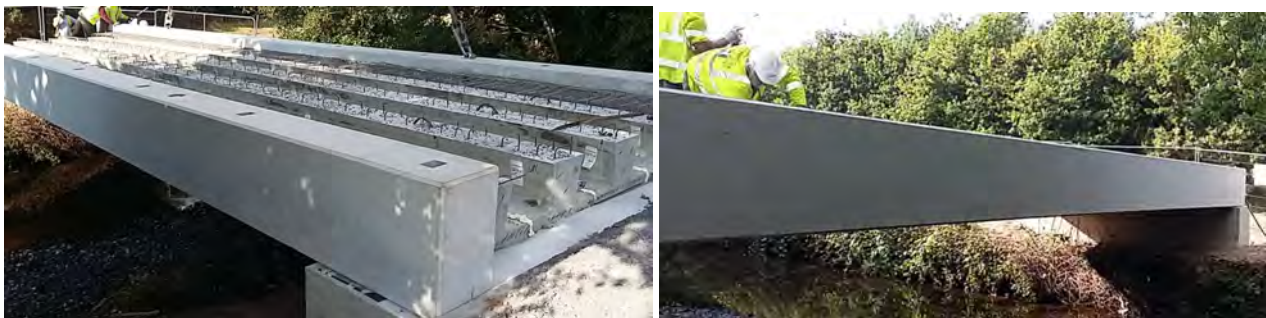
Figure 4.16: Economical precast prestressed concrete bridge beam option for approach ramp elevated structure (southern approach ramp)
