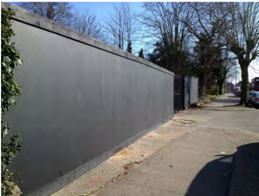
Image 6: Example of suitable hoarding
