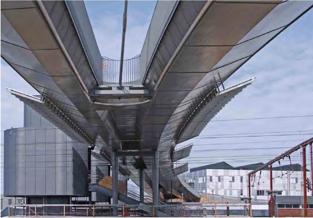
Figure 11 Example of under bridge screening on new pedestrian and cycle bridge in Odense, Denmark with 1.2m high parapets with vertical bar infill
