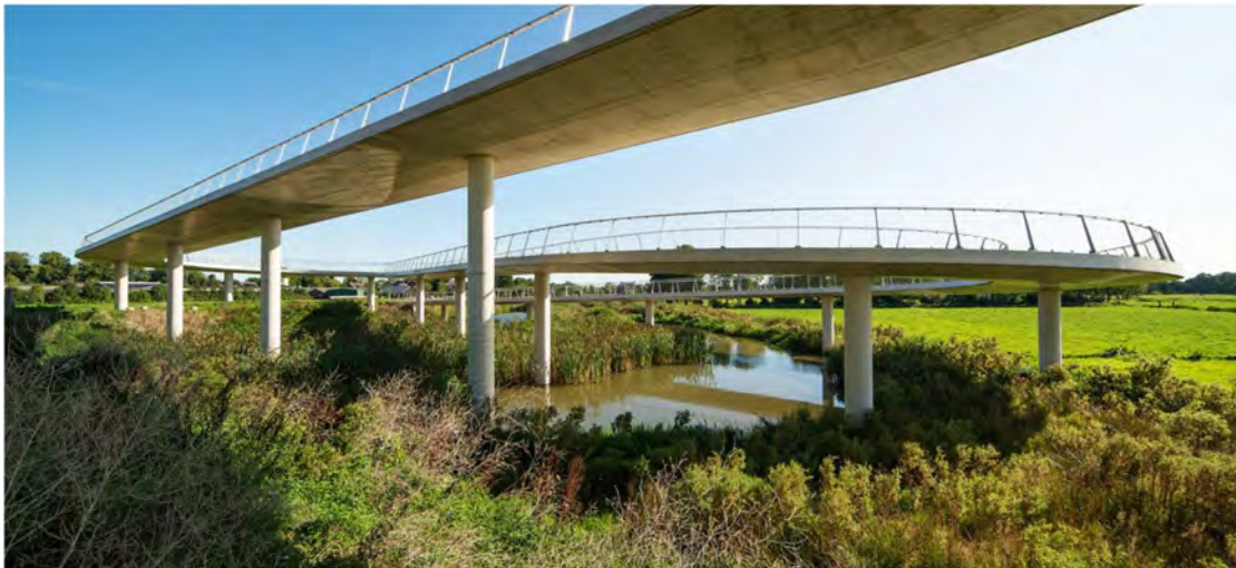
Figure 4.15: Example of reinforced concrete elevated ramp structure with monopiles/columns (northern approach ramp)
