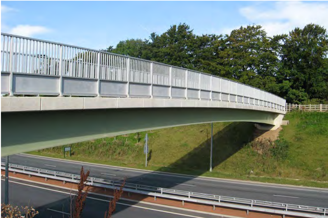
Figure 15: Double Span Through Girder
