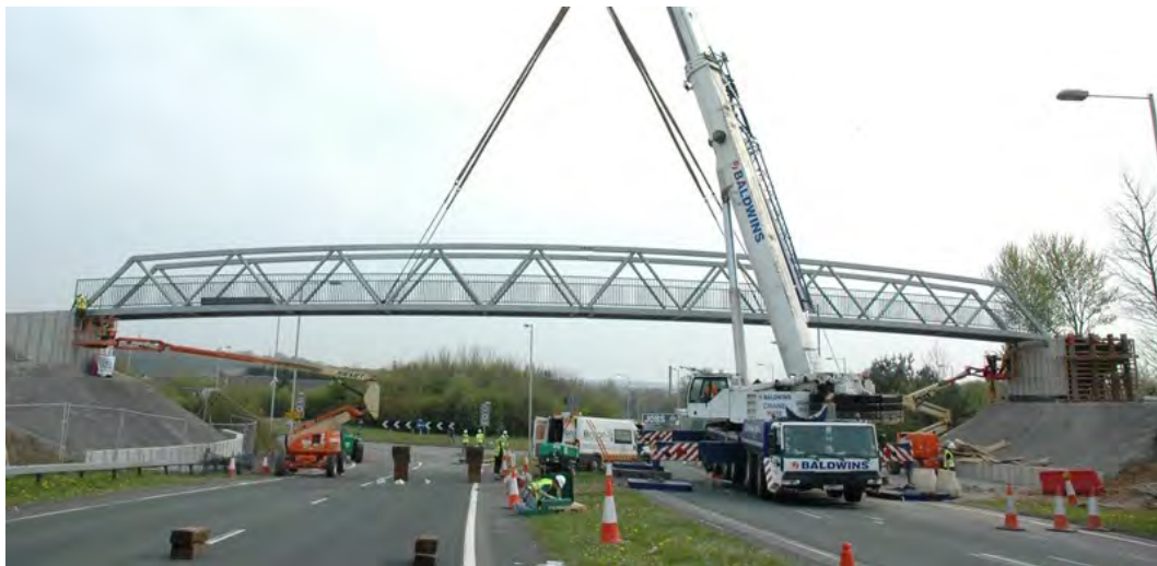
Figure 20: Bridge Erection during Road Closure
