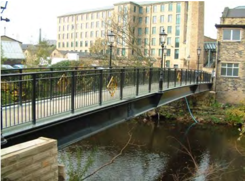
Figure 4.13: Steel edge beam bridge
