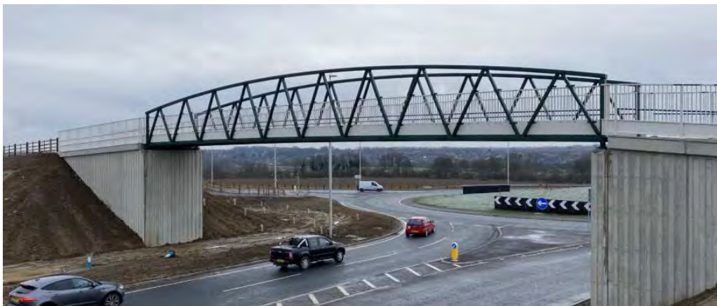
Figure 4.7: Example of shorter span steel through truss over road
