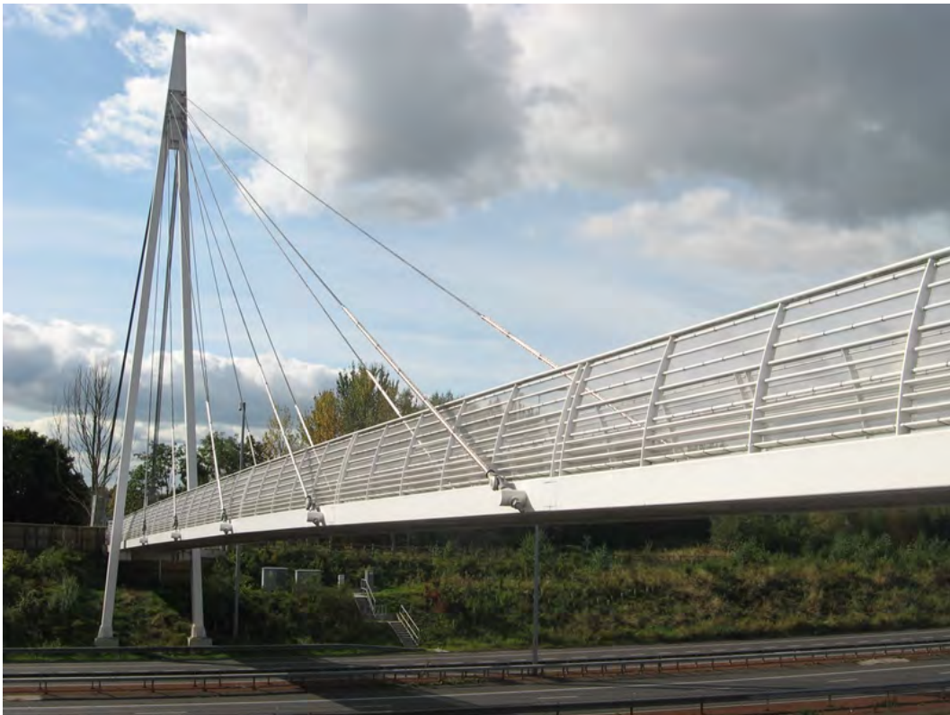
Figure 19 Cable Stayed Bridge Example
