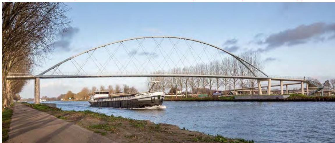
Figure 4.9: Example of steel network arch pedestrian and cycle bridge with concrete deck
