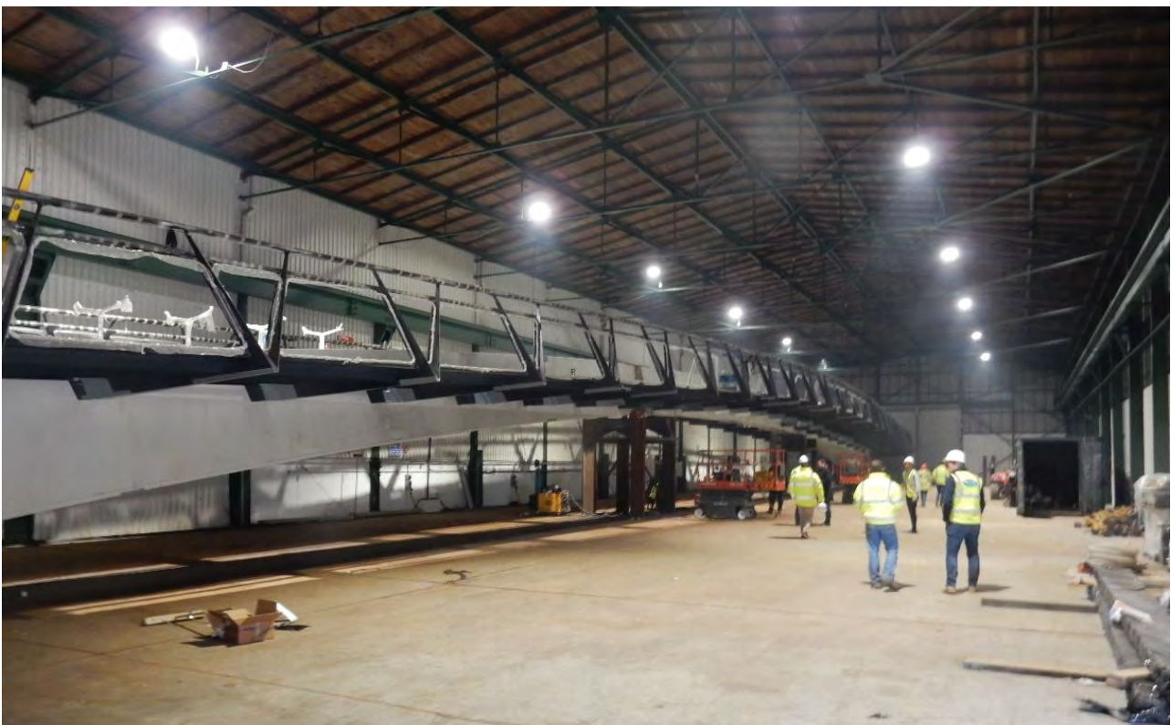
Image 5.7: Example of bridge fabrication and pre-assembly in workshop
