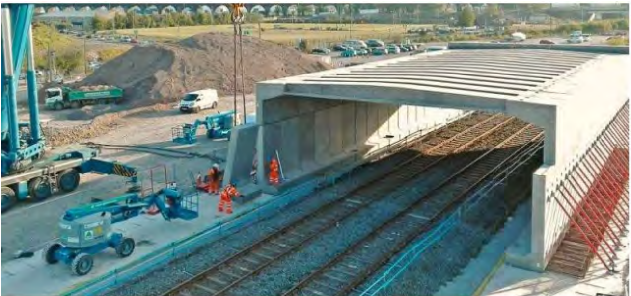
Image 3.13: Example of segmental precast reinforced concrete porta frame structure over rail
