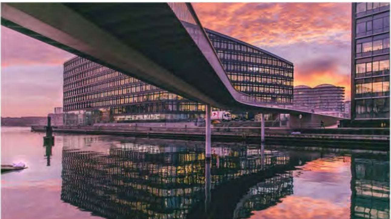
Image 3.15: Example of steel elevated ramp / cycleway structure with spine beam and monopiles / columns
