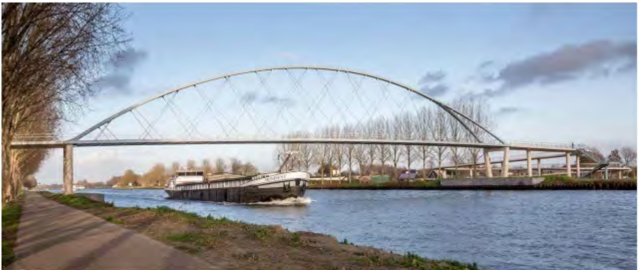
Image 3.12: Example of steel network arch pedestrian and cycle bridge with concrete deck
