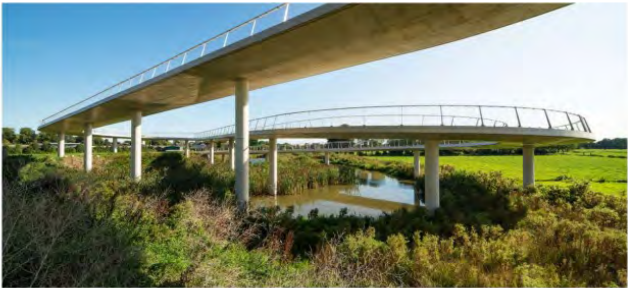
Image 3.18: Example of reinforced concrete elevated ramp structure with monopiles / columns (northern approach ramp)
