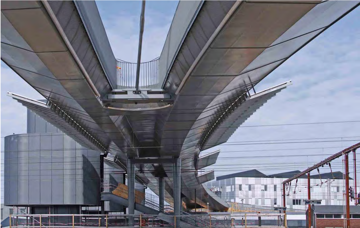
Image 4.27: Example of under bridge screening on new pedestrian and cycle bridge in Odense, Denmark with 1.2m high parapets with vertical bar infill
