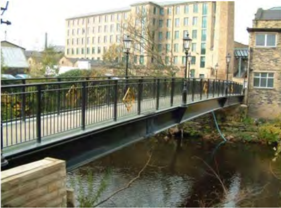
Image 3.16: Steel edge beam bridge
