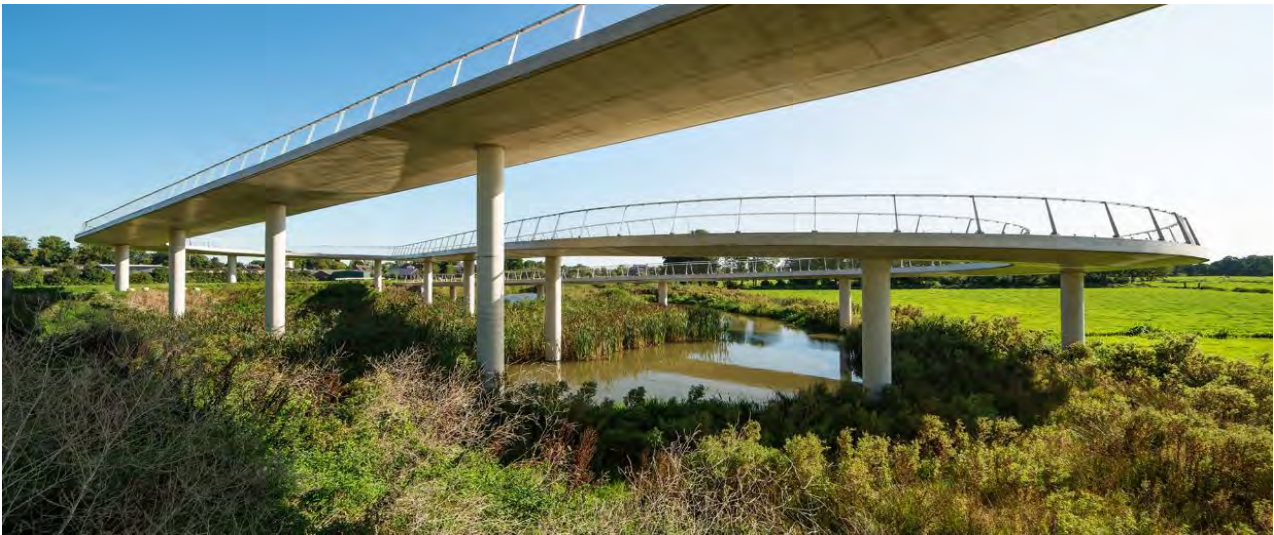
Image 4.21: Example of reinforced concrete elevated ramp structure with monopiles / columns (as proposed for the northern approach ramp)
