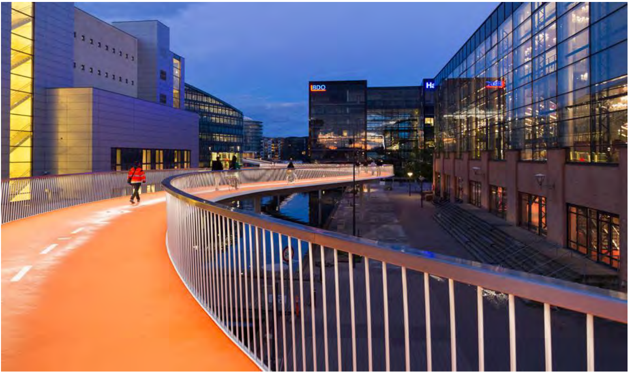
Image 4.26: Parapet type with vertical parapet infill
