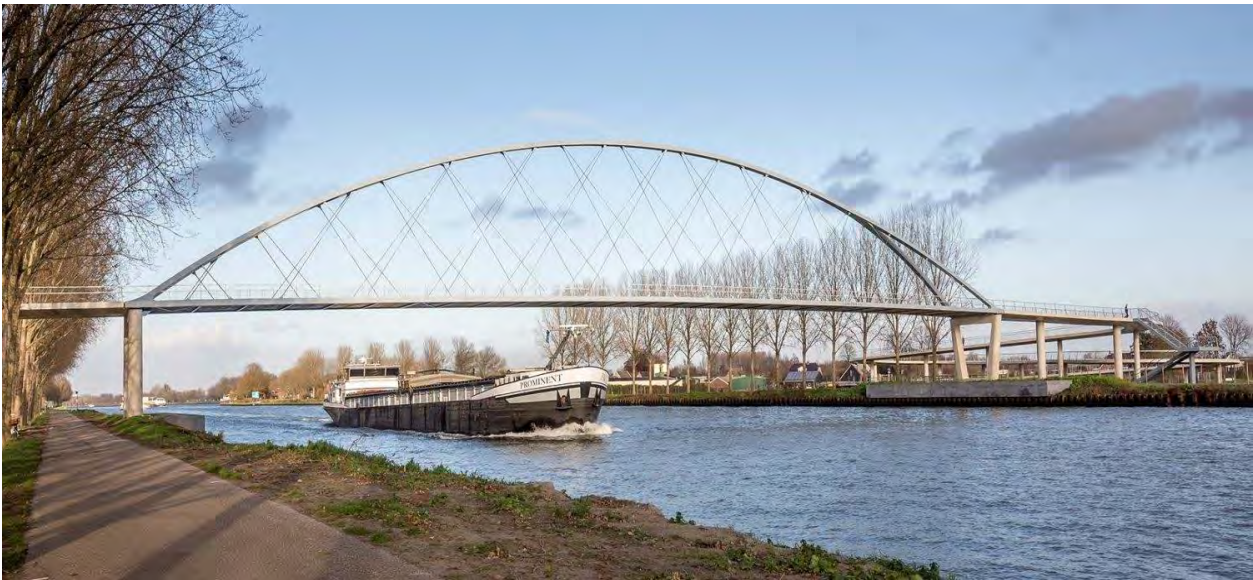
Image 4.18: Example of steel network arch pedestrian and cycle bridge with concrete deck
