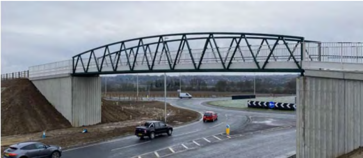
Image 3.10: Example of shorter span steel through truss over road
