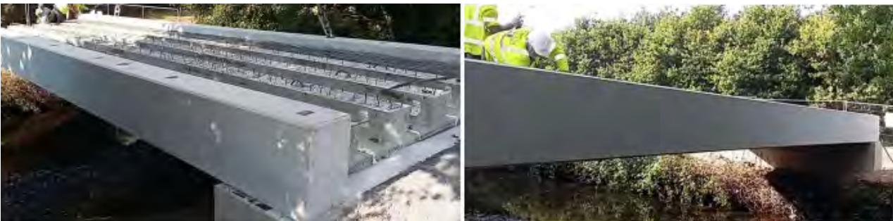
Image 3.19: Economical precast prestressed concrete bridge beam option for approach ramp elevated structure (southern approach ramp)
