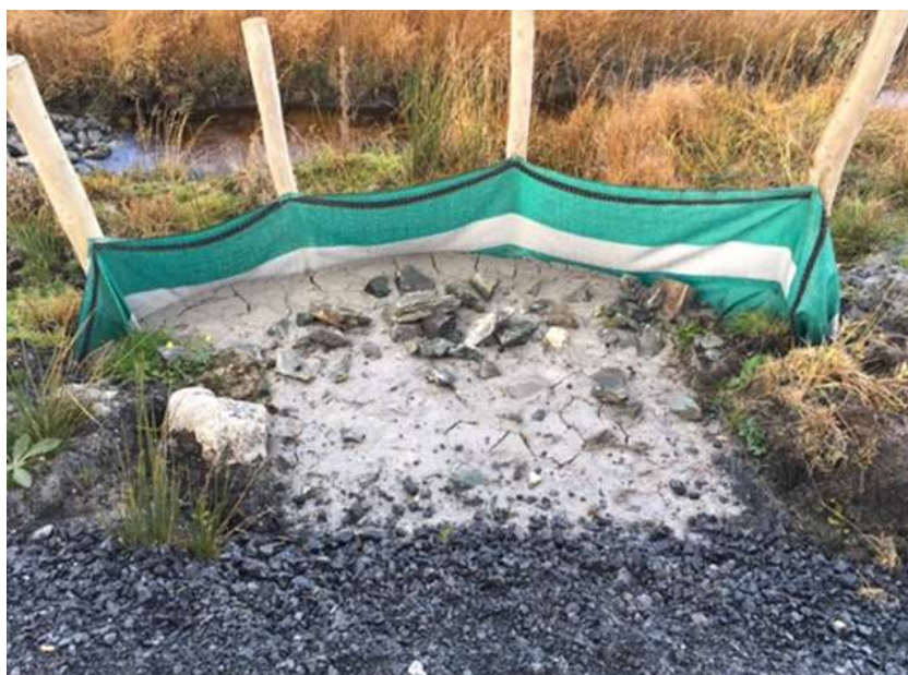
6-2 Fabric Silt Fencing Protecting Water Course
