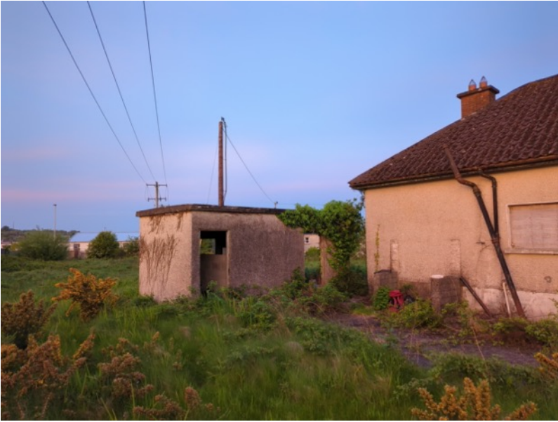
Plate 3. Small storage shed close to dwelling. Open draughty concrete block with concrete ceiling and flat roof. Very low potential for roosting bats
